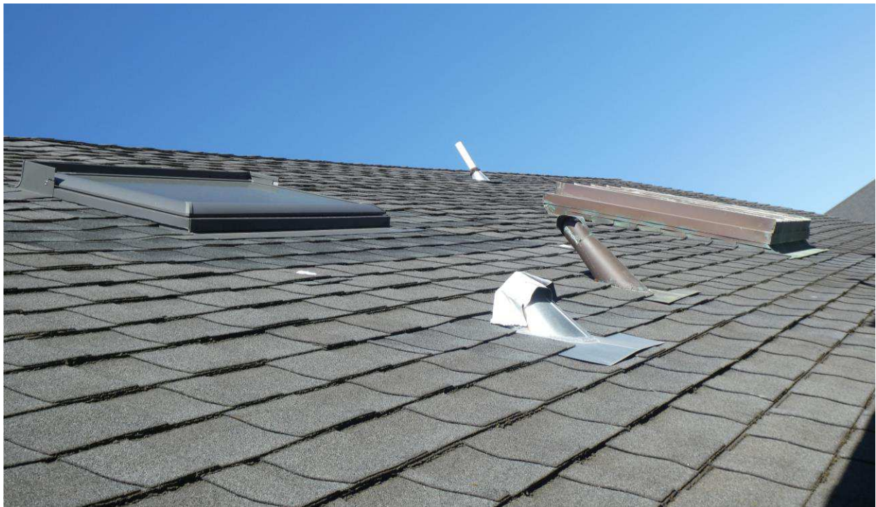
Figure 53: Detail of the asphalt shingle roofing on the main roof and two skylights. The original copper skylight over the interior stair is to the right in the photo.
