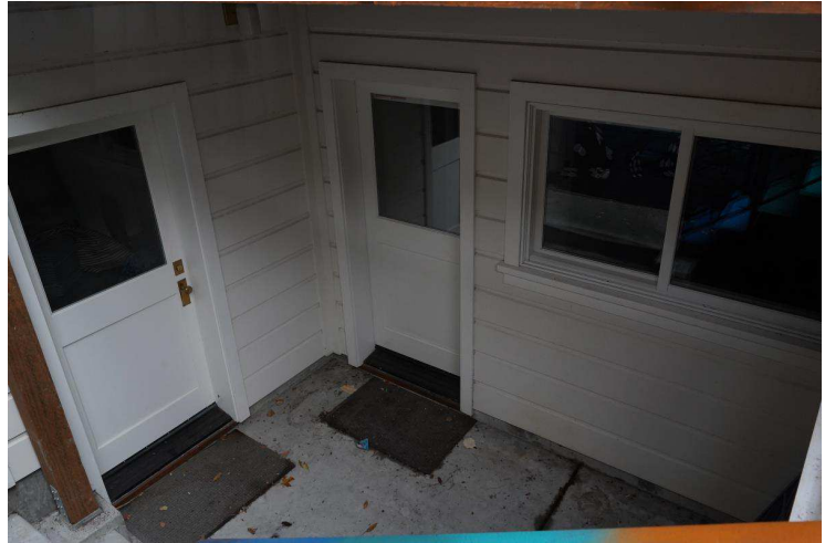
Figure 16. Basement doors and windows at rear of building, view north.
