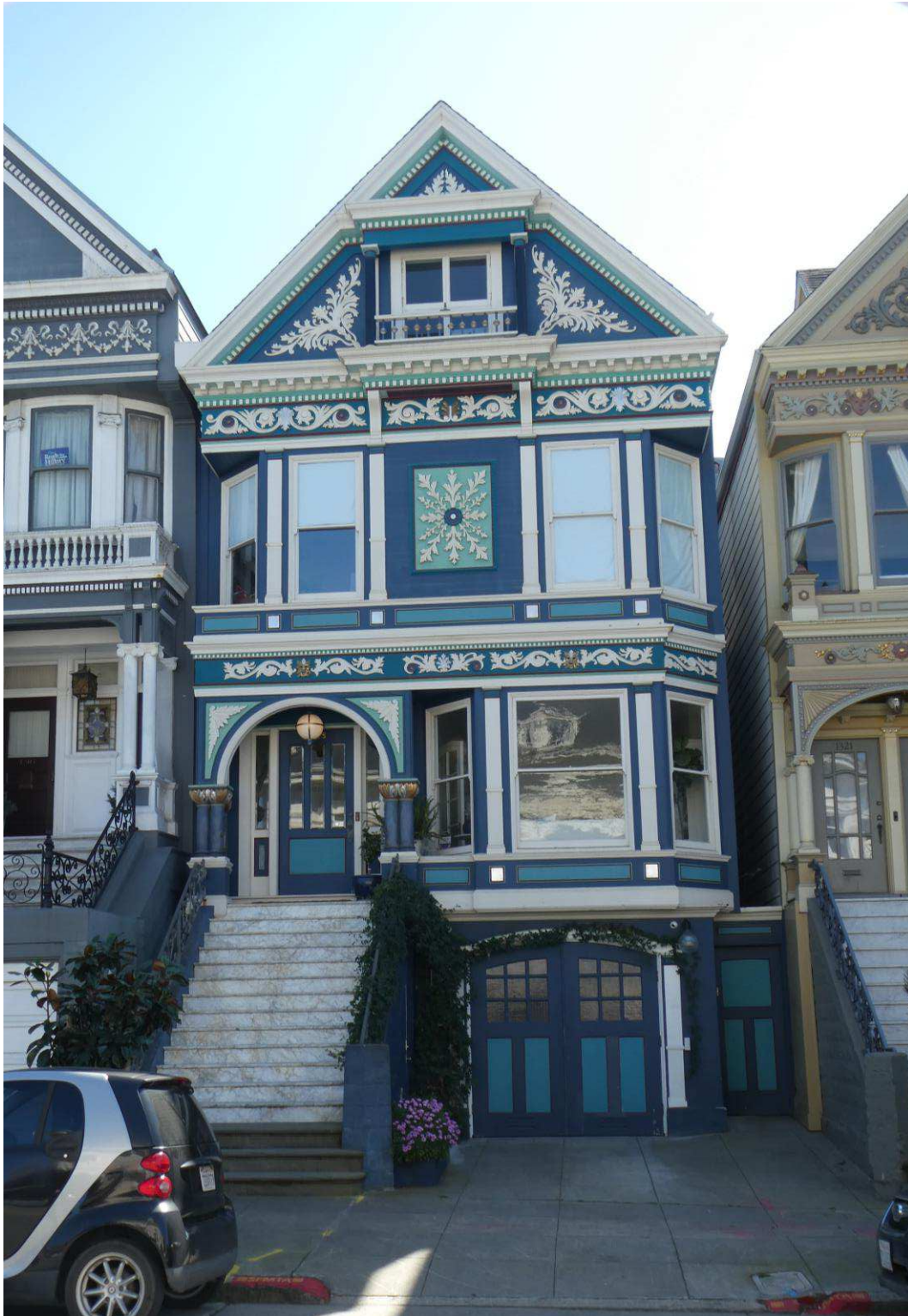
Figure 26. Front northwest façade, view southeast.
