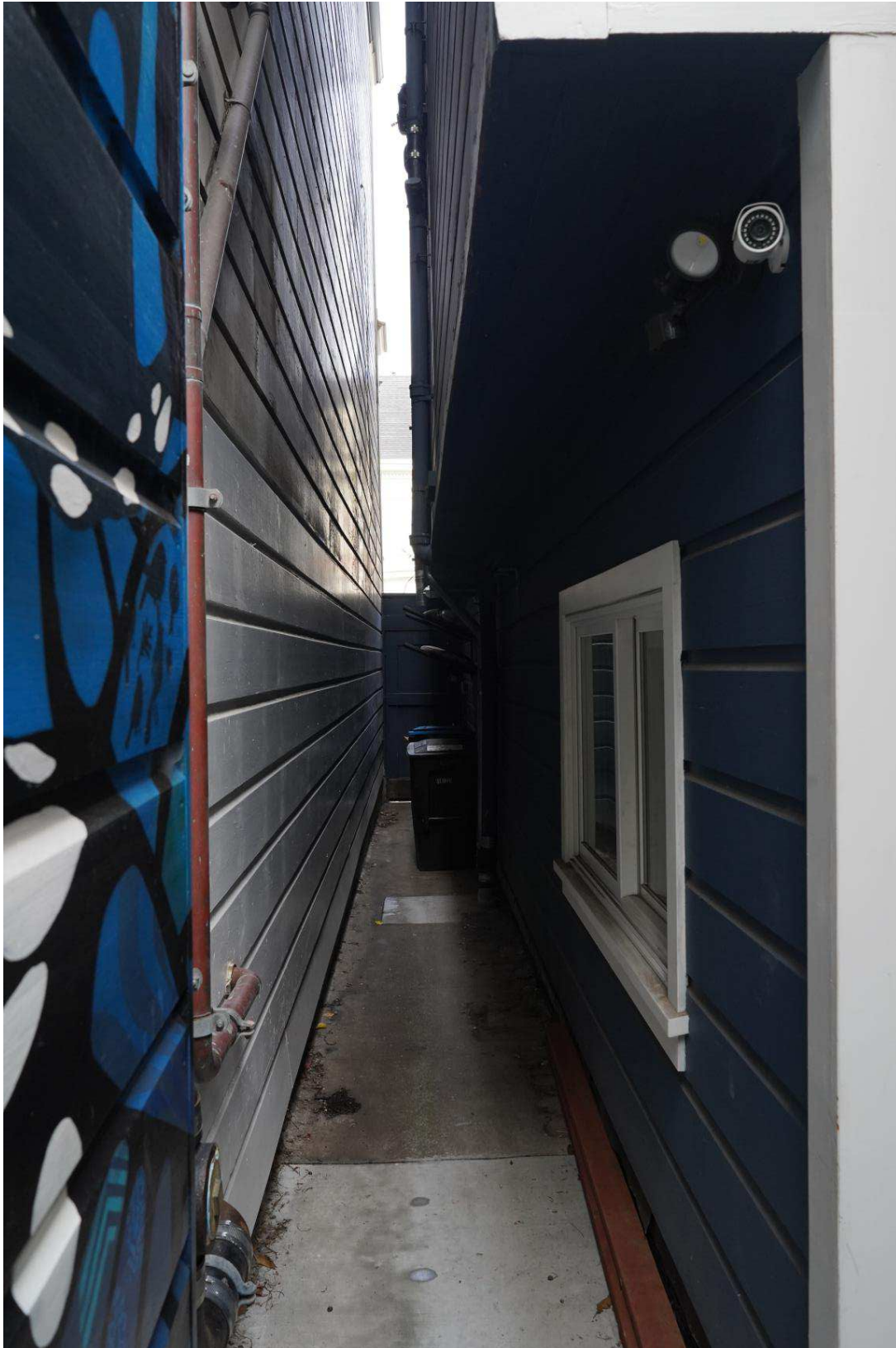
Figure 31. Southeast façade at basement level, view northwest.
