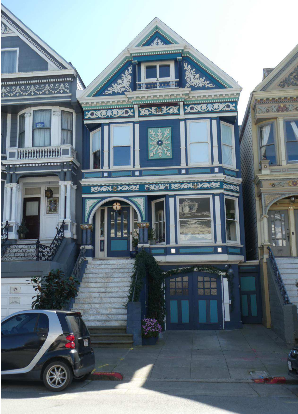
Figure 24: Overall photo showing the primary Waller Street Façade.
