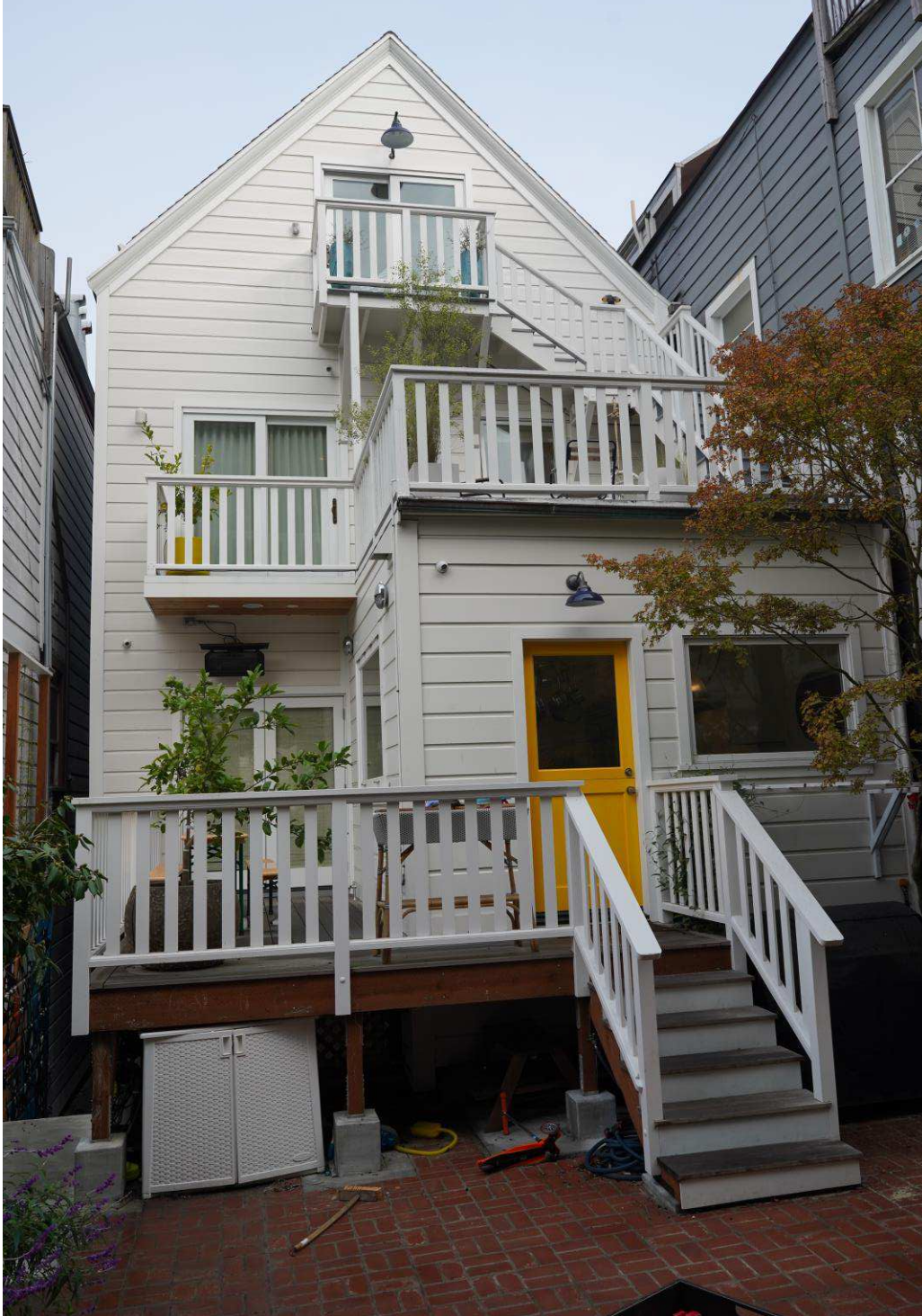
Figure41. Overall view of the rear, southeast facade, view northwest.
