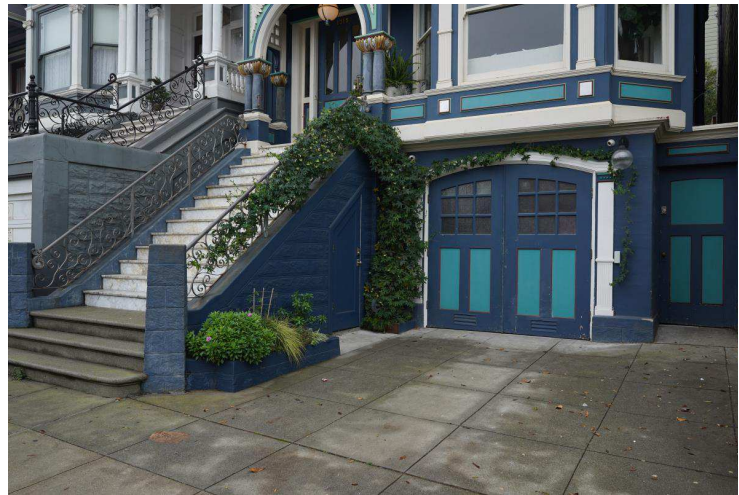
Figure 12. Garage and exterior front stairs at northwest facade, view southeast.
