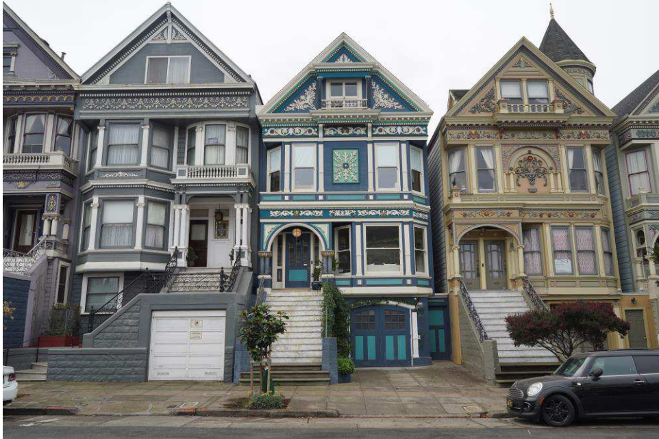
Figure 2: 1315 Waller Street, primary facade, November 2019. Looking southeast.
