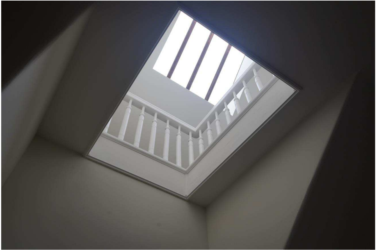
Figure 51. View looking up at the third-floor stair landing and skylight.
