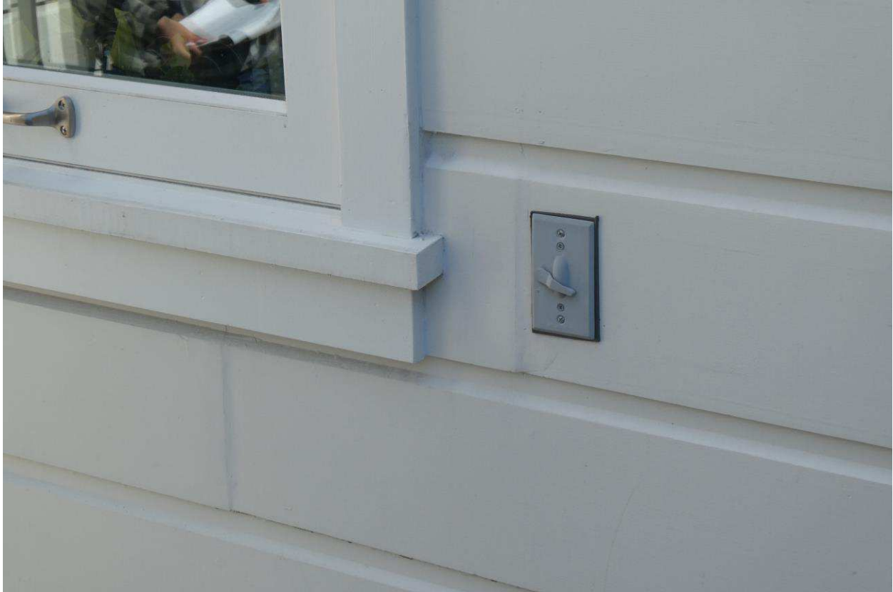
Figure 45: Detail of bulging siding at the lower corner of the window, southwest side of the first floor kitchen.
