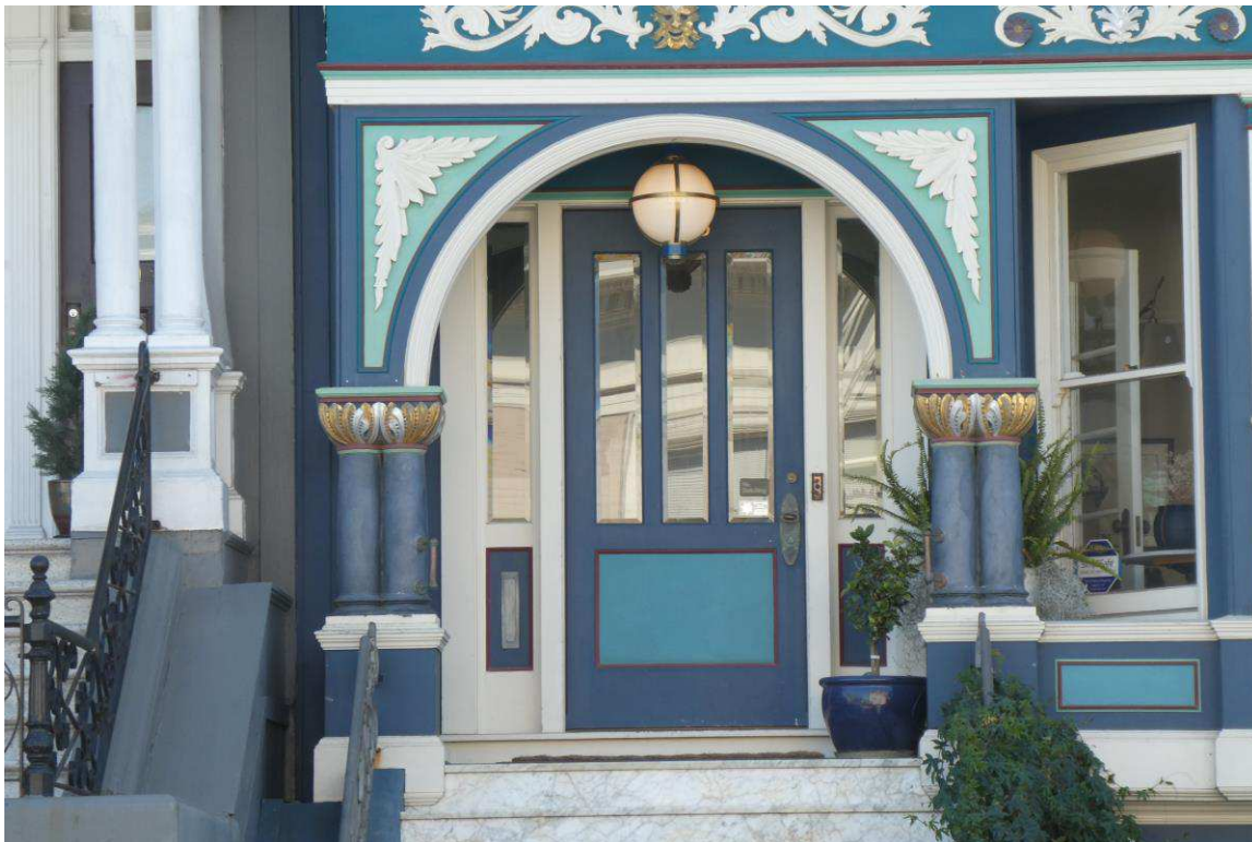
Figure 28. Front entry detail, view southeast.
