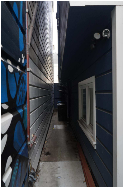
Figure 17. Southeast façade at basement level, view northwest.
