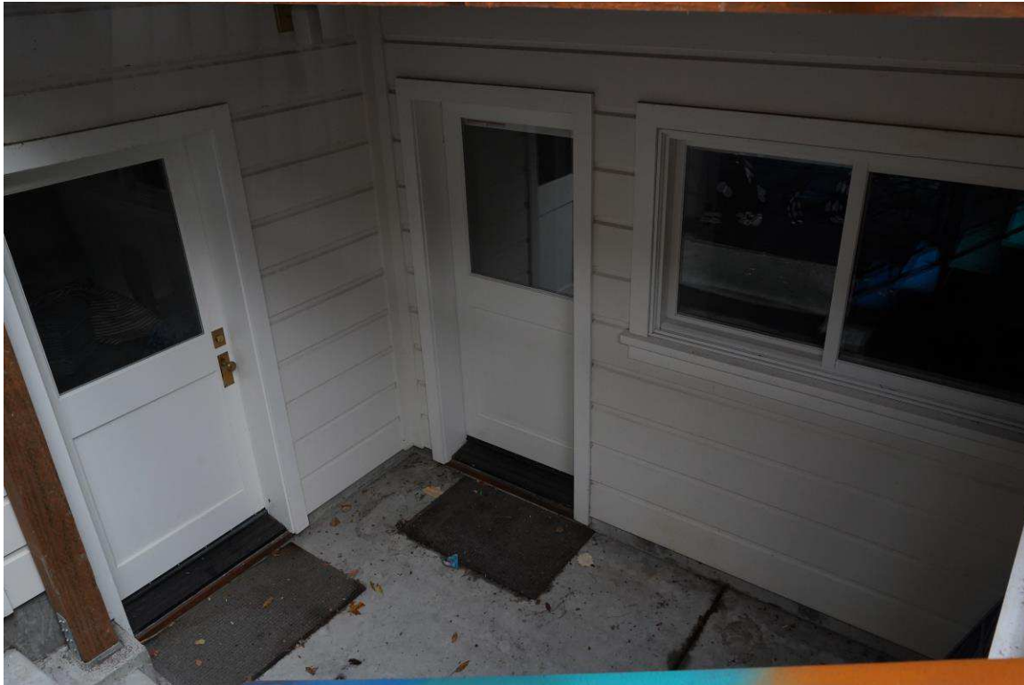
Figure 32. Basement doors and windows at rear of building, view north.
