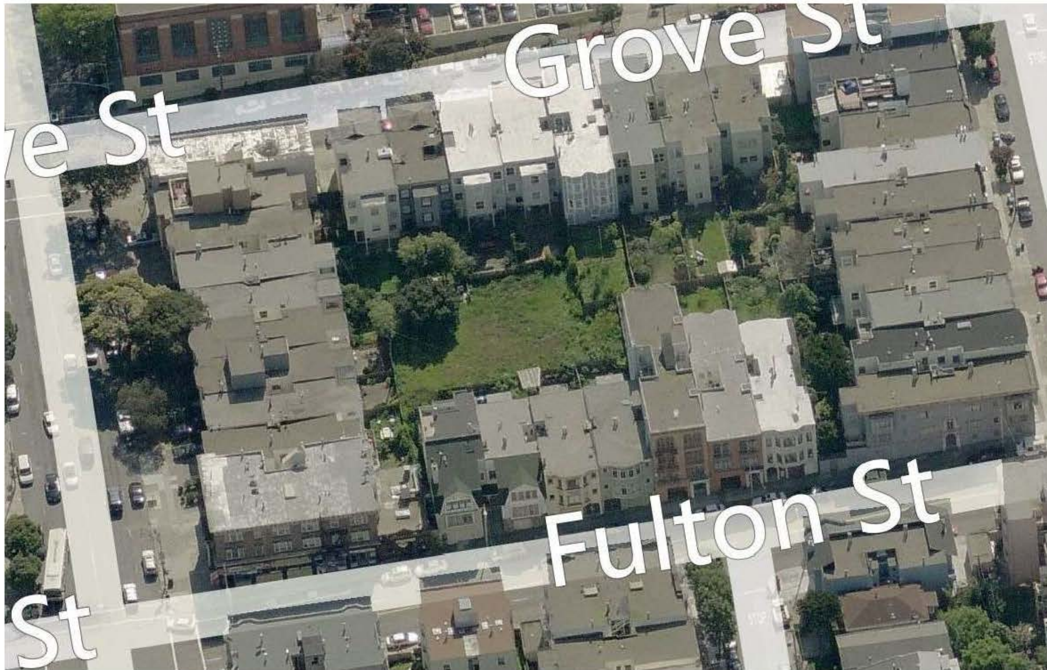
Overhead View of Site
