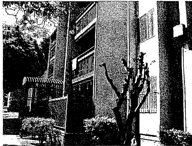
EXTERIOR VIEW OF SUBJECT
