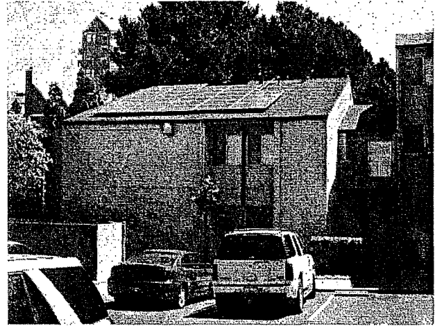
EXTERIOR VIEW OF SUBJECT
