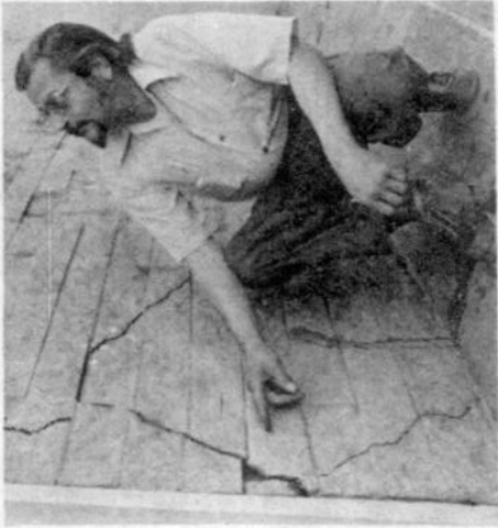
CUSTODIAN JOHN CASE CHECKS CRACKS IN WALL Structure is moving sideways and down at same time
