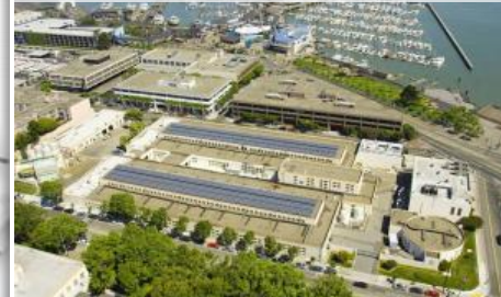
North Point Wet Weather Facility
