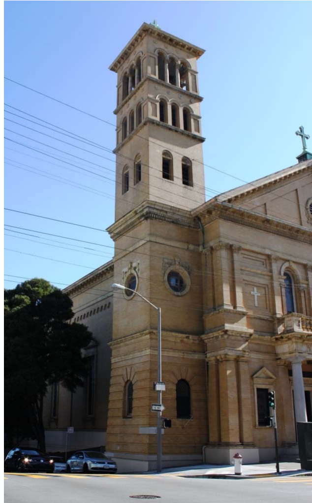
FIGURE 7. CHURCH: CAMPANILE, LOOKING SOUTHEAST FROM FILLMORE ST., 2015.
