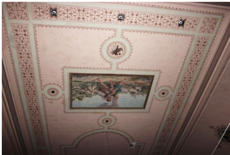
FIGURE 29. CHURCH: NAVE, WEST PORTION OF PAINTED CEILING, 2016.
