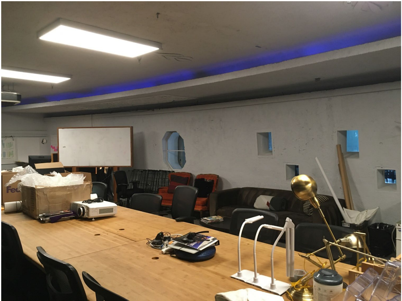
Grand Theater, second floor interior addition with original rear wall of auditorium and holes in wall for projection booth, 2023. Source: SF Planning Department
