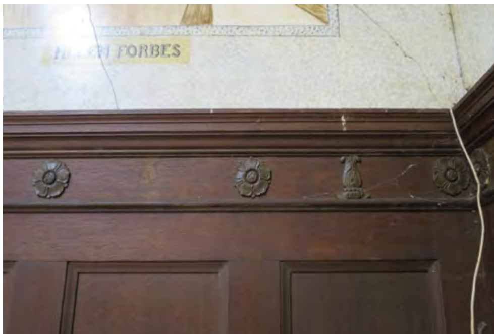
Mother's Building, detail of metal motifs at wainscoting in main lounge, 2016.
