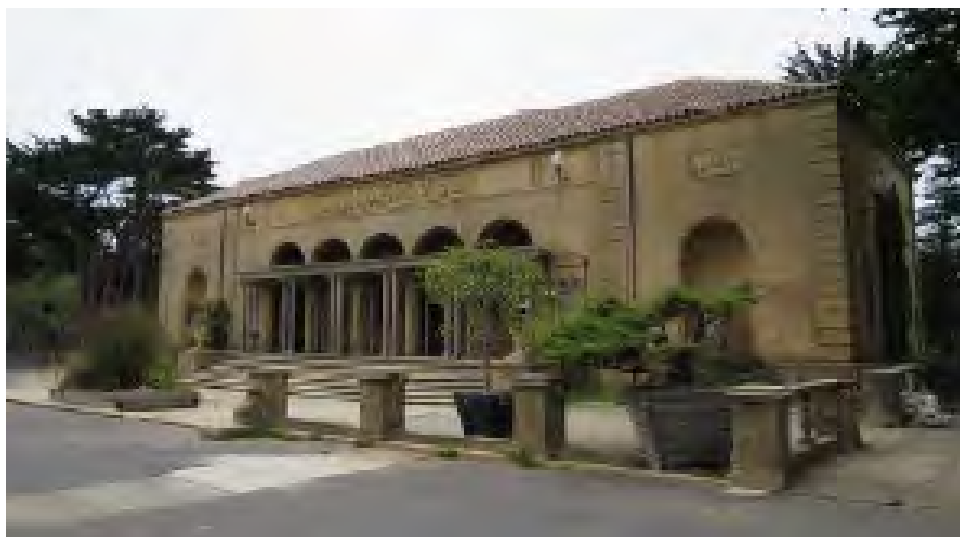
Mother's Building, east elevation and terrace/plaza, view southwest, 2015. Source: SOHA Engineers
