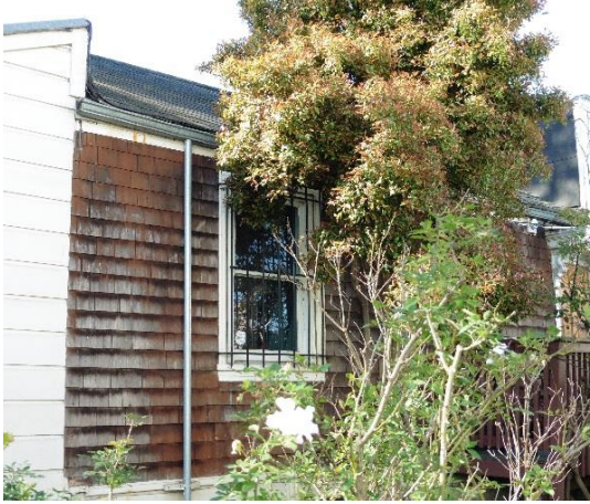
Figure 11. Double hung window at north façade, looking southwest.
