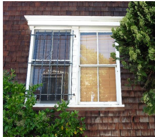
Figure 6. Primary façade windows.
