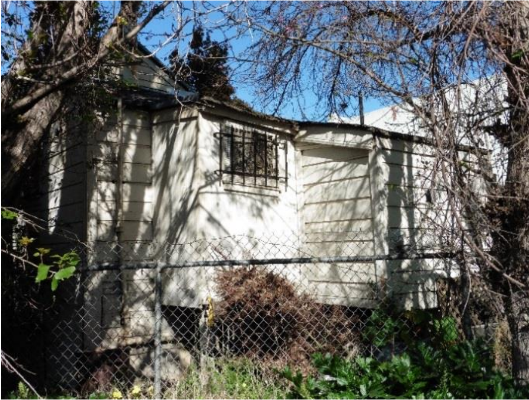
Figure 15. Projecting volumes on north portion of facade, looking northwest.
