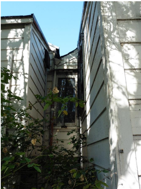
Figure 16. Window at center of building, looking west between two projecting volumes.
