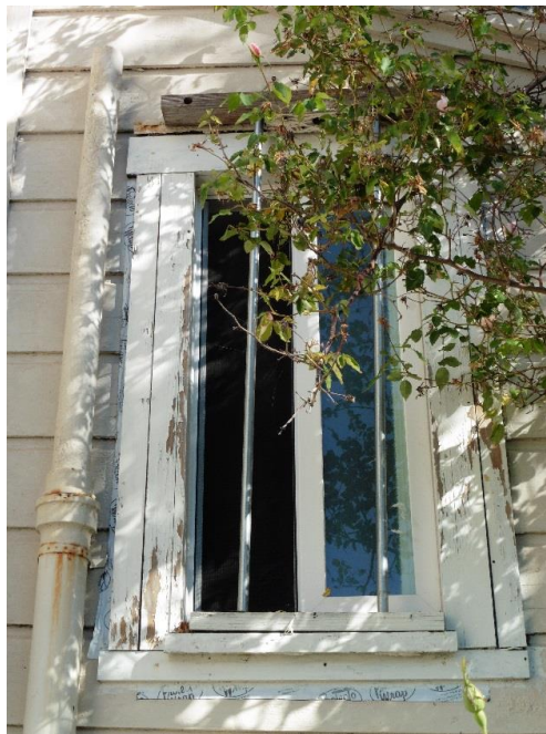
Figure 20. Vinyl window within wood frame on south side of projecting addition.
