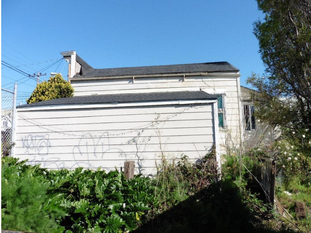
Figure 21. South façade, looking north.
