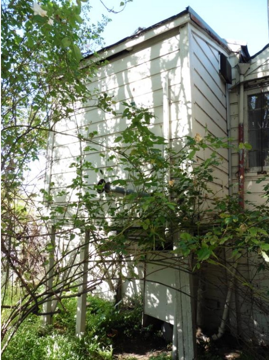
Figure 18. Projecting volume at south portion of façade, looking south.
