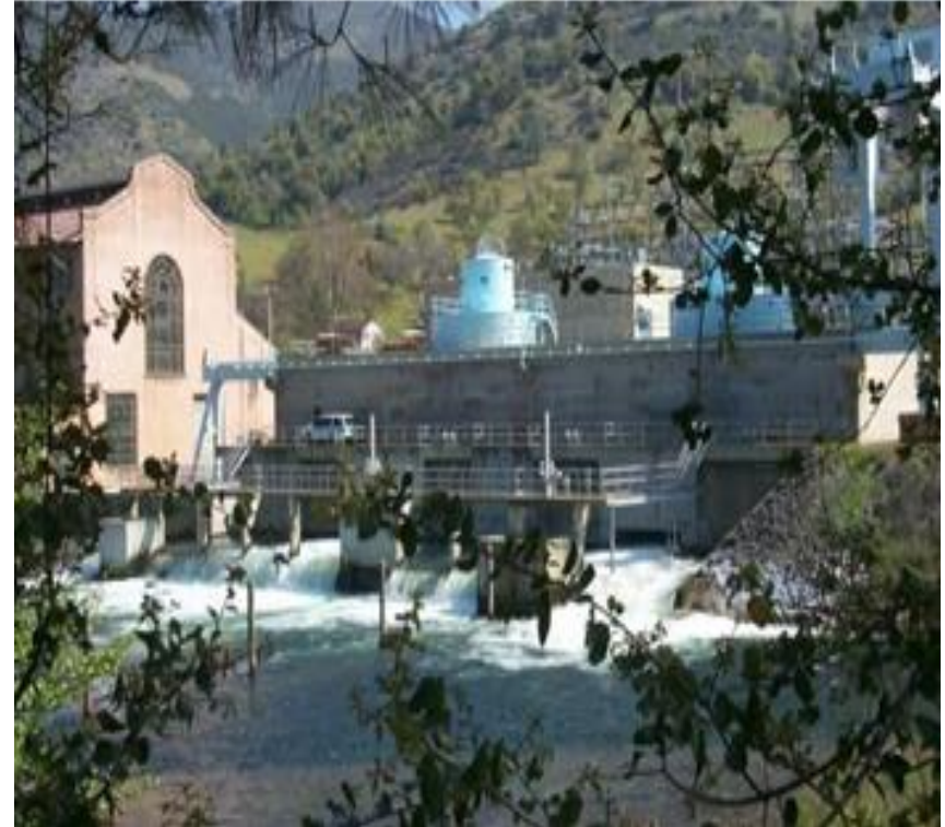
Moccasin Power House
