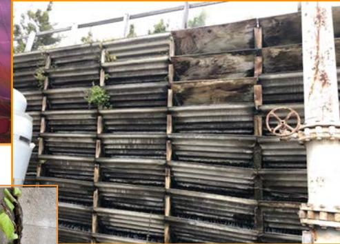
Cooling Tower failing structure (above) and rusted out sump (below)
