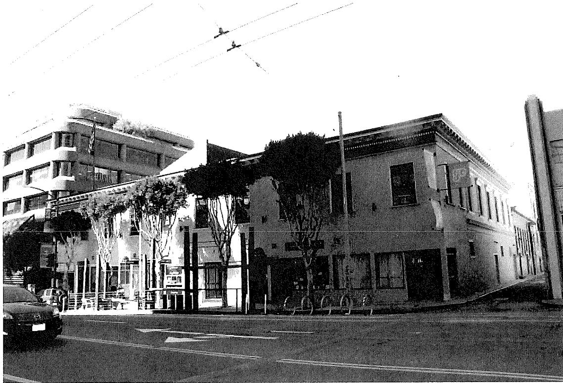
Primary elevation, view west.
