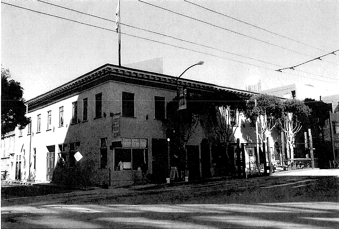
228-248 TOWNSEND STREET NEW PULLMAN HOTEL
