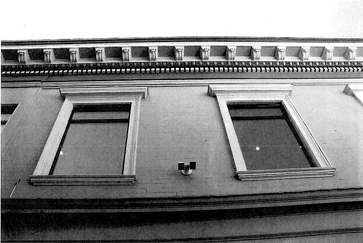
Window detail on Clyde Street elevation, view west.
