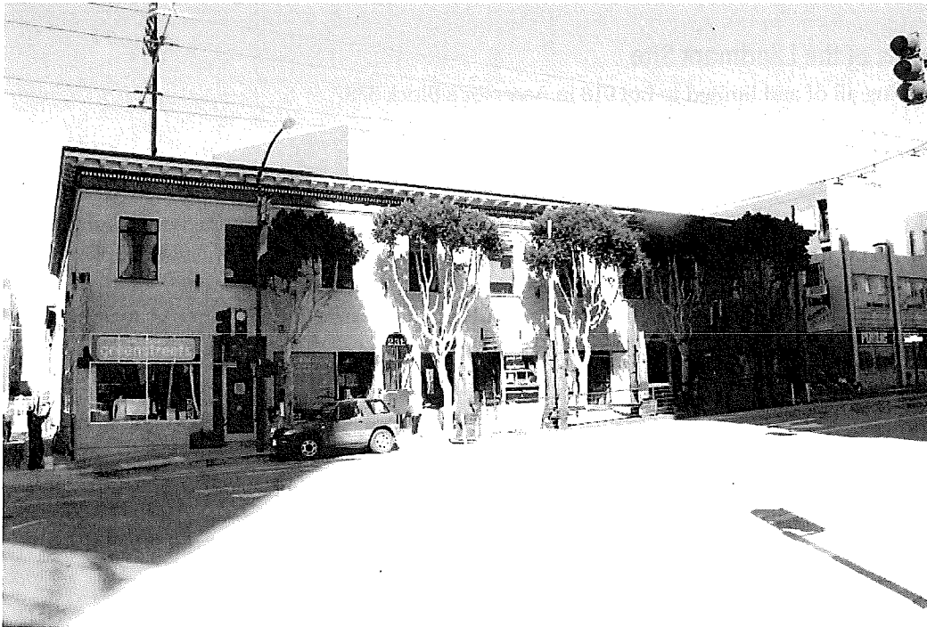
Primary elevation, view northwest.
