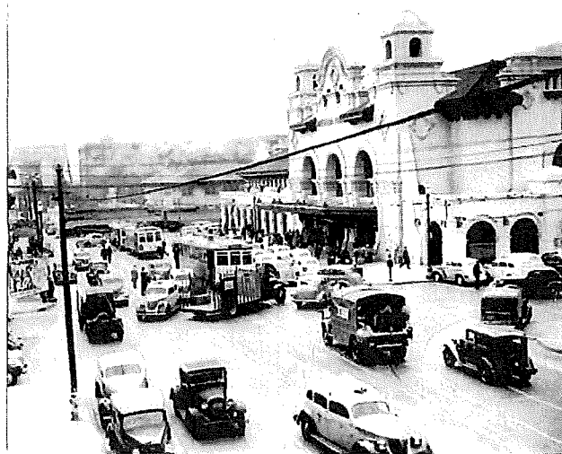
Southern Pacific Depot, 3 rd and Townsend Streets, June 16, 1939 (San Francisco Public Library)
