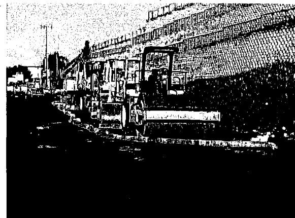
Inactive paving equipment is properly stored with perimeter protection.
