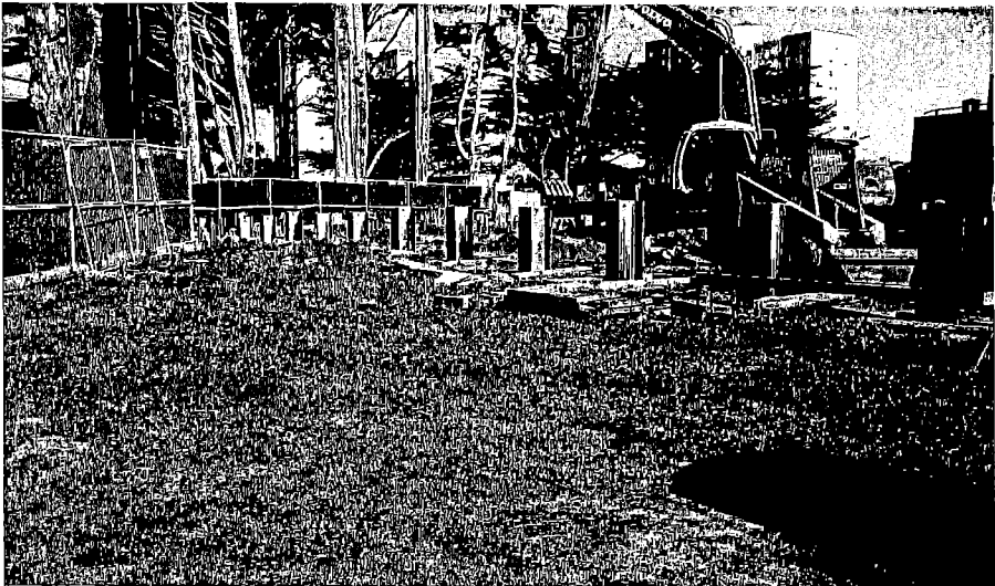
Extend the silt fence to the top of the perimeter fencing. This provides wind control and site security.
