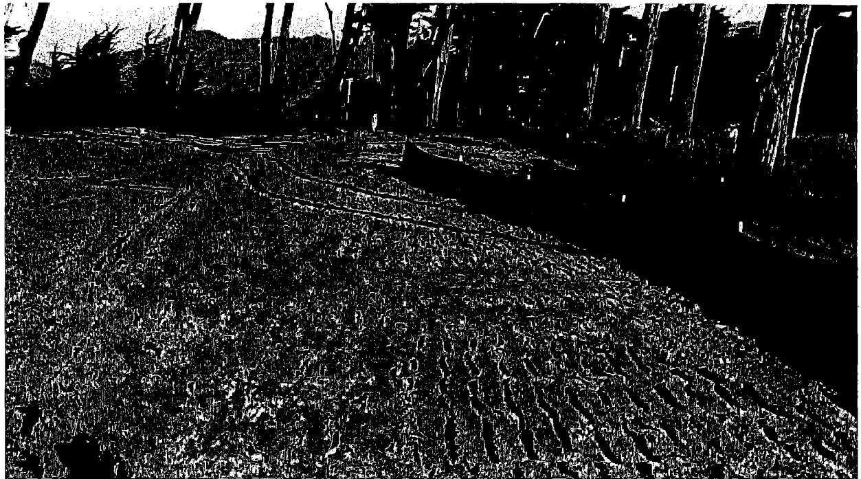
Soil roughening can be used as a complementary process for controlling erosion.
