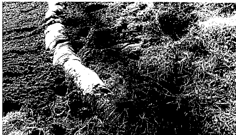
Straw mulch is applied to help vegetation establishment.
