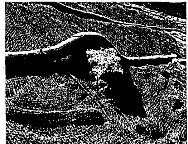
Remove or by pass all obstructions prior to placing fiber roll. Do not install the roll over the obstruction.
