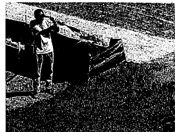
A hydraulic mulch with binder is applied to a disturbed soil area.
