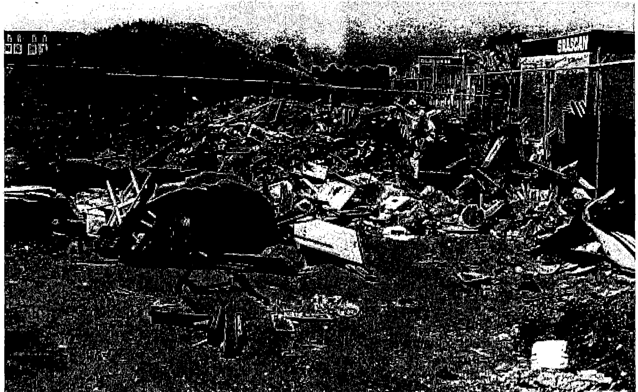
Illegal trash dumping on a construction site.
