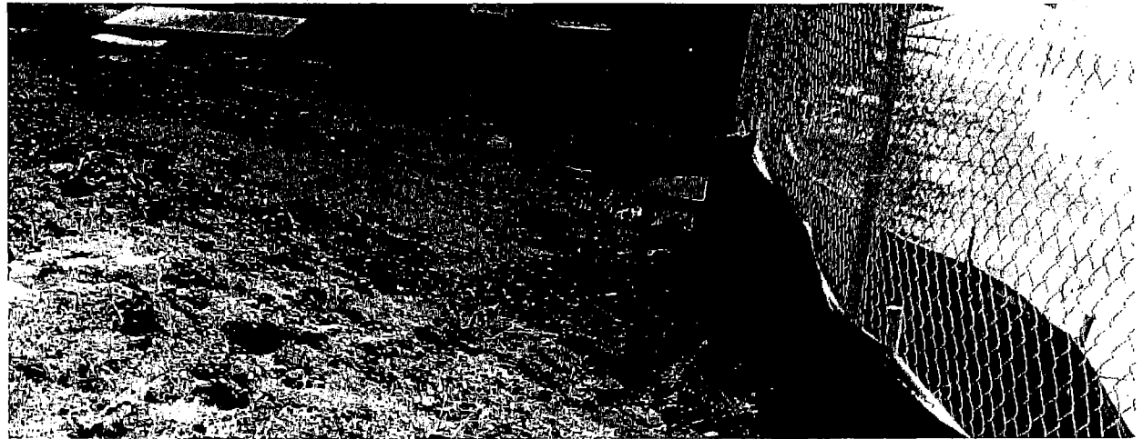
Silt fence is attached to construction fencing to prevent sediment from leaving the site.
