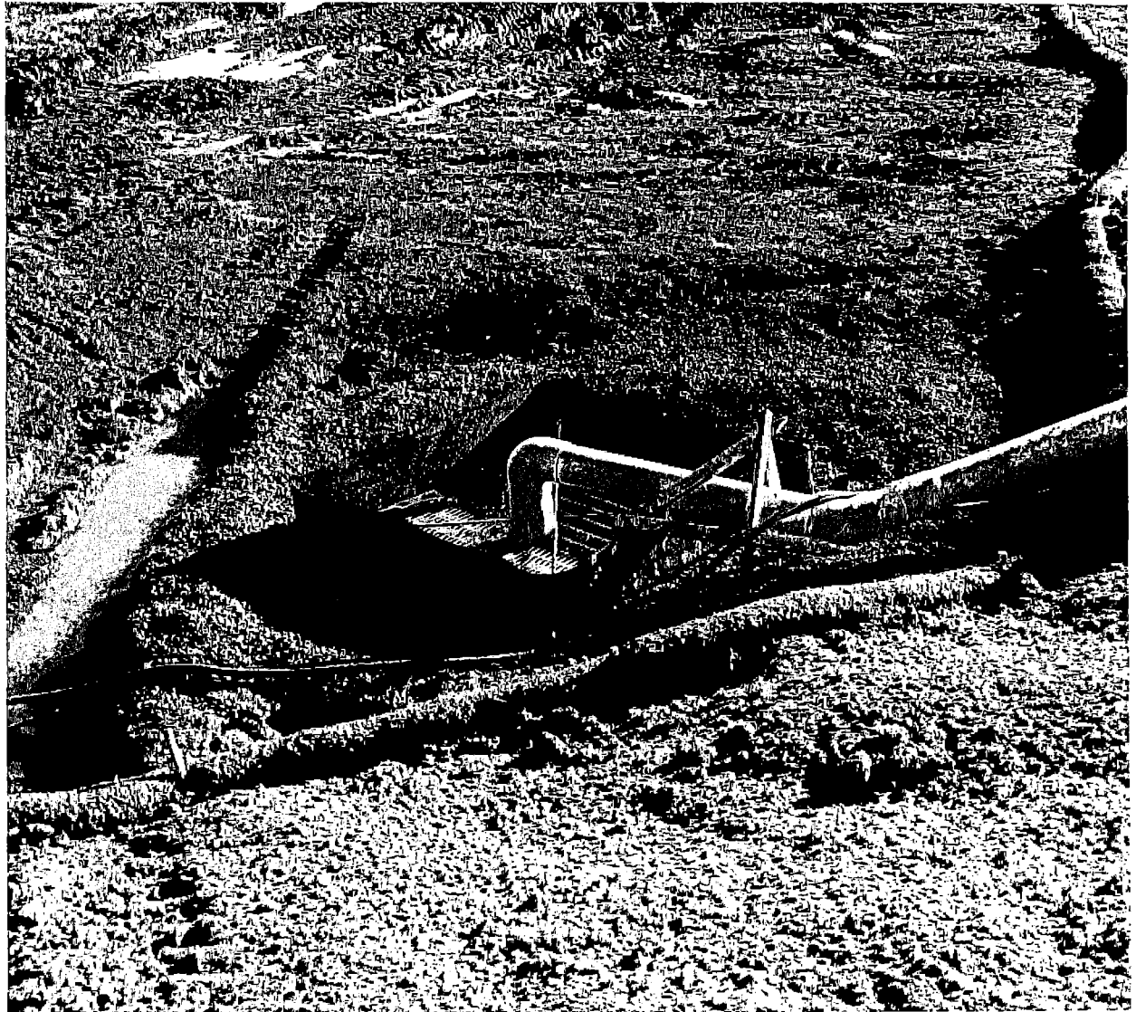
Clean runoff is directed to the storm system through a slope drain. This prevents the runoff from flowing down the steep slope.
