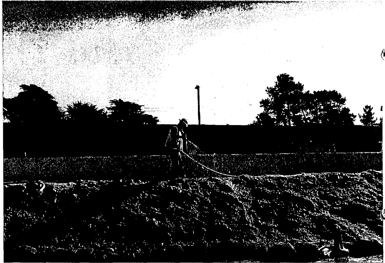
A construction worker is applying a bonded fiber matrix to disturbed soil area.
