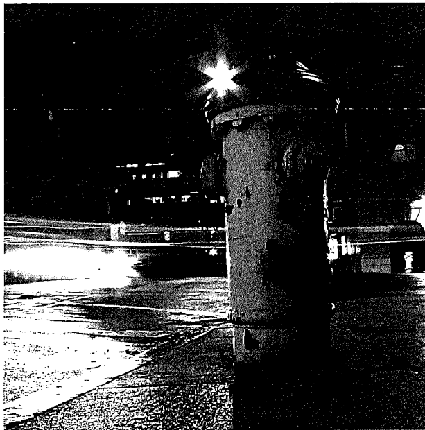
High Pressure (AWS) Fire Hydrant. Photo by Flickr user fivein1/13716 .
