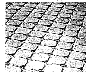
Required saw-cut joints
