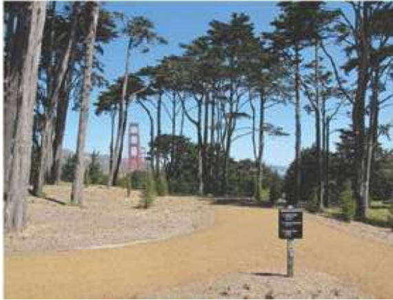
STABILIZED AGGREGATE PAVING
