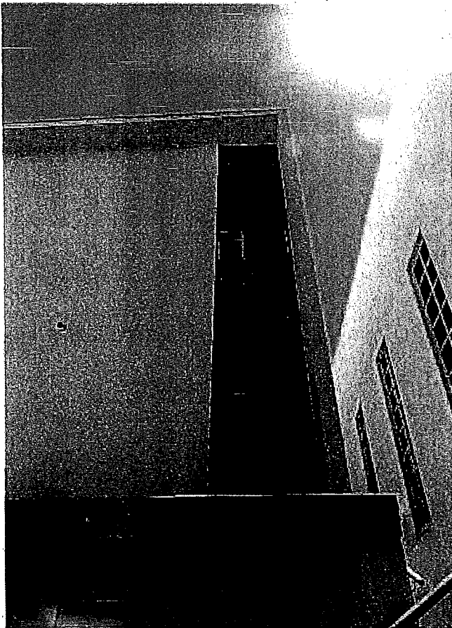
Vertical wood ribbon windows with textured yellow glass on north elevation of youth center and fellowship building, view south.
