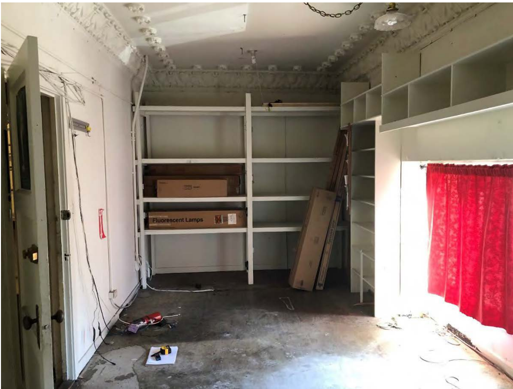
Clay Theatre, Second Floor office, room was created in 1946 remodel so ceiling moldings may date from original construction, 2020 Source: DNM Architecture
