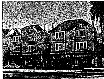
Examples of significant breaks
