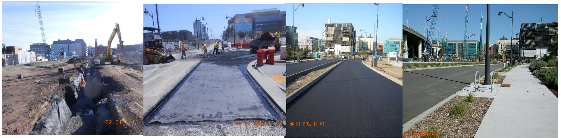
Utility pipe installation and active street paving through final landscape
