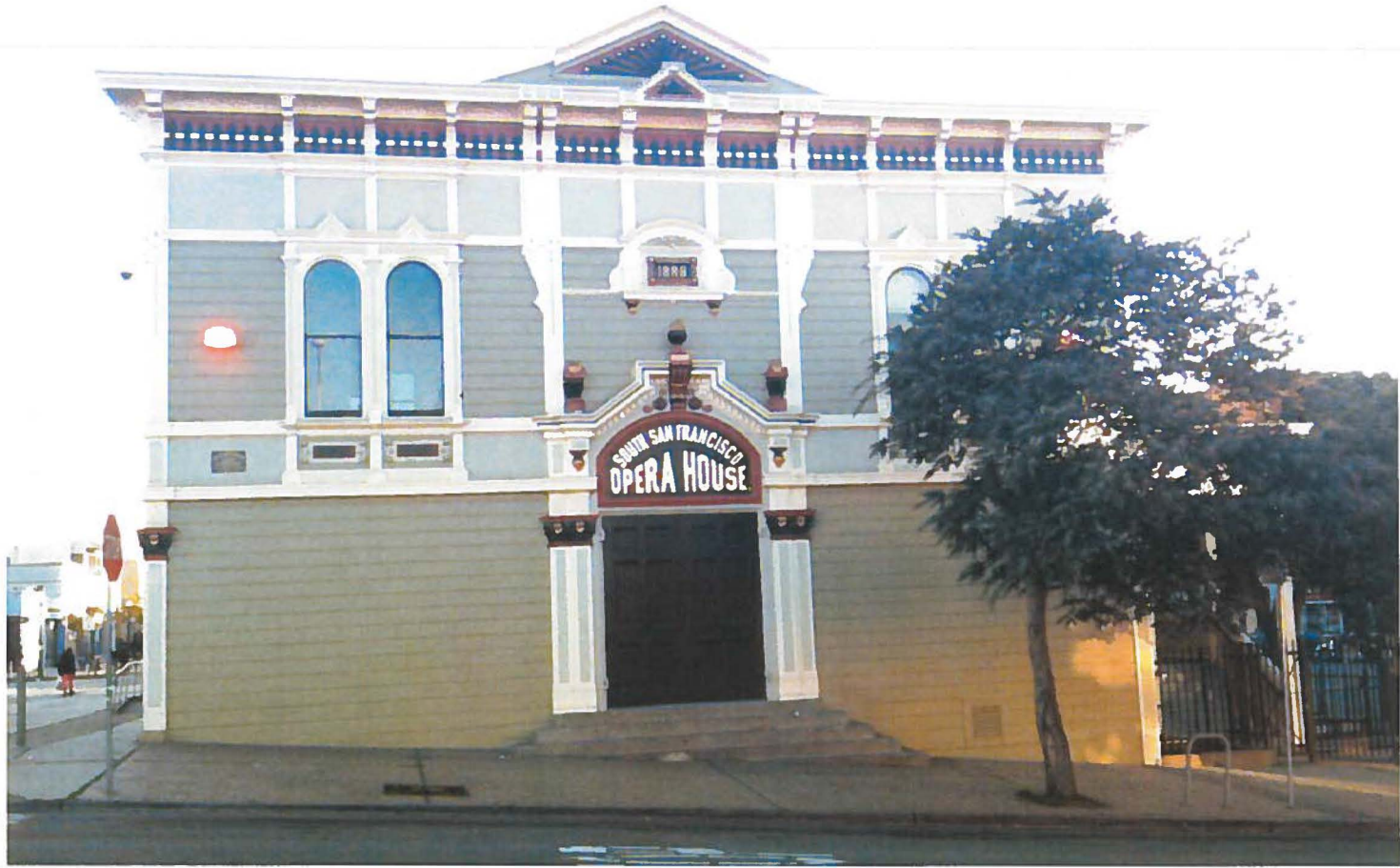
EXISTING MAIN ENTRY
