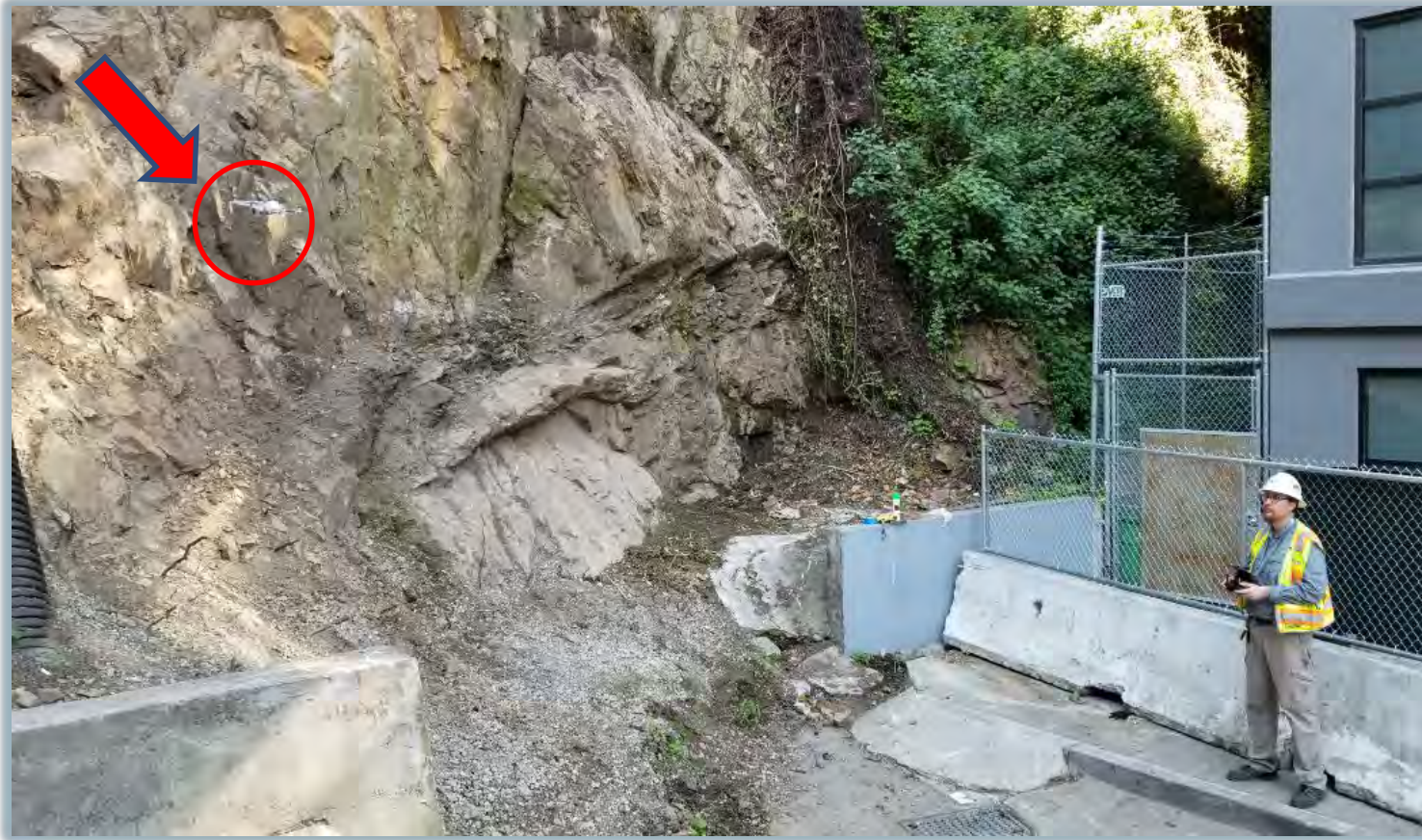
Photo: Filbert Street hillside inspection, 2019
