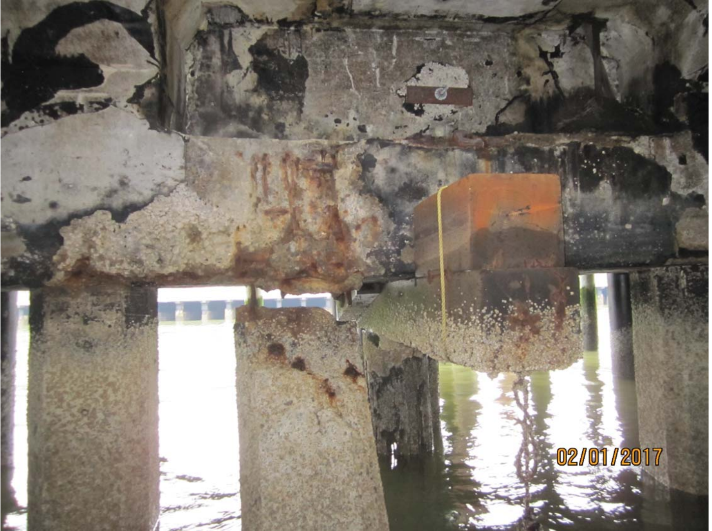
Photo 10. Conditions inside northern edge of pier. Many batter piles are broken in the north-east quadrant of the pier. Broken batter piles do not affect gravity load capacity of pier.
