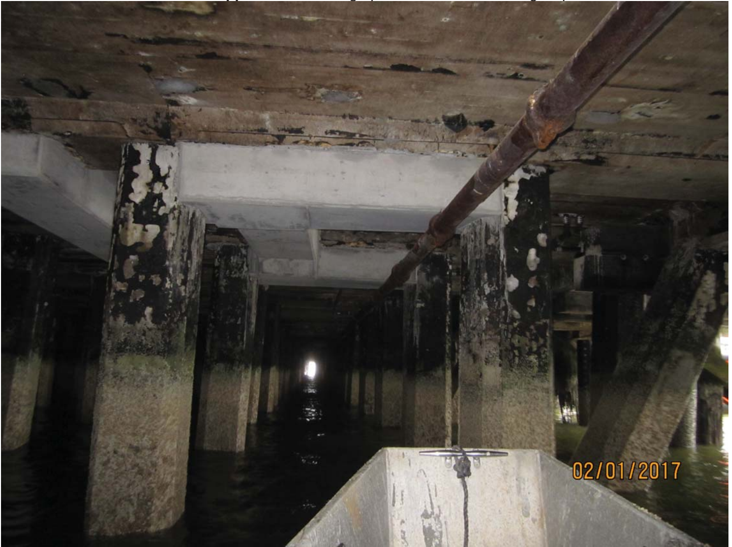
Photo 13. New concrete beams added along near south edge of pier. Could not locate drawings for this work.
