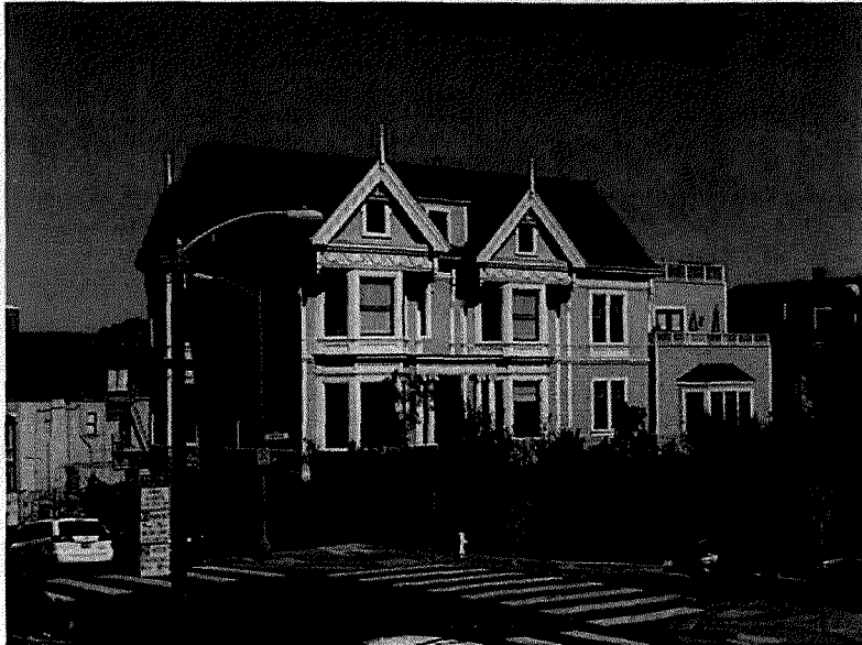
Figure 1. Overall view of 940 Grove Street, looking northeast (Garavaglia Architecture, Inc., October 2016)
