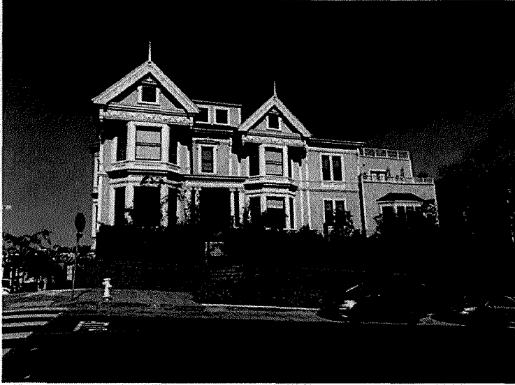
Figure 12. View 940 Grove Street's south facade along Grove Street (Garavaglia Architecture, Inc., October 2016)
