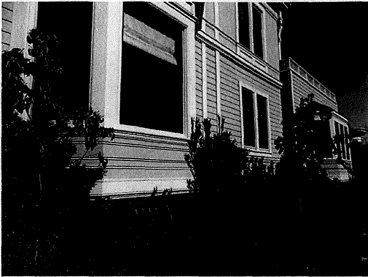
Figure 10. View 940 Grove Street's three types of wood siding along the south facade of the house, with different siding found above the raised basement, at the first floor, and at the upper floors (Garavaglia Architecture, Inc., October 2016)
