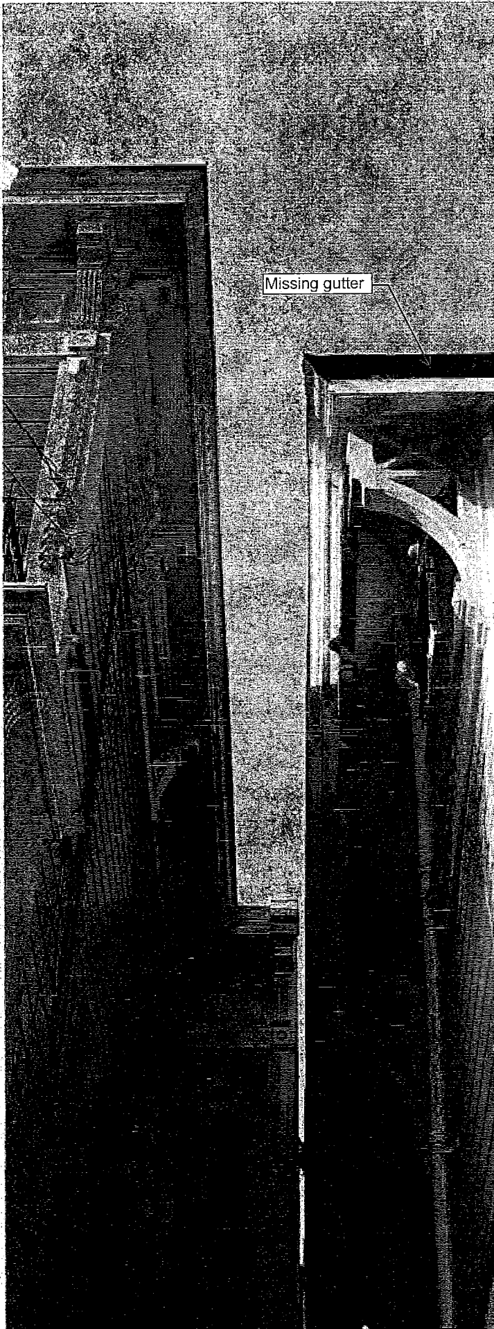
Close up: Proximity of eaves to adjacent property.
