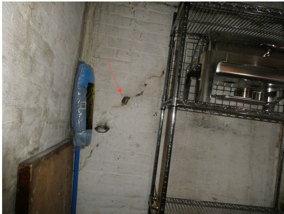
Figure 59: Detail view of the diagonal crack, south basement wall.
