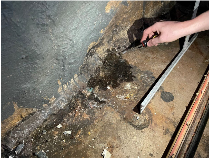
Image 27: View of typical area of water intrusion at west foundation wall, basement floor. (Photo taken by P&T 03/14/2025)
