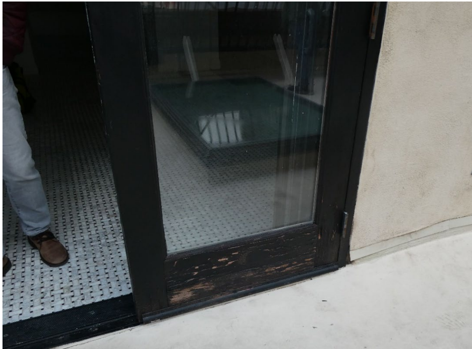
Figure 29: Deterioration of the bottom rail of the glazed doors, south façade.
