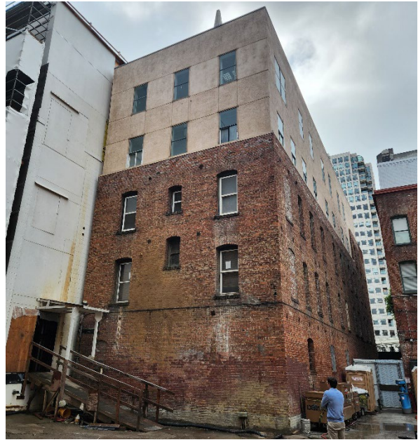
Figure 11: Rear of 530 Jackson Street, 2025. Note the two-story addition, visible with stucco exterior above the original brick exterior. Source: Page & Turnbull.
