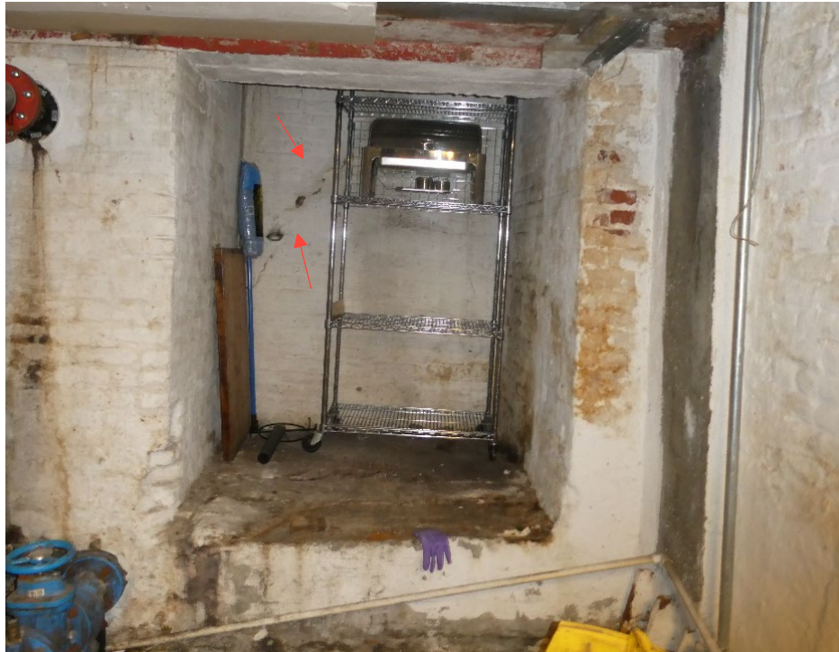
Figure 58: Diagonal crack in the south basement wall under the sidewalk hatch.
