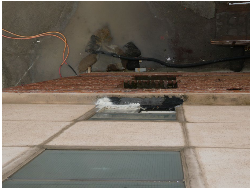
Image 14: North facade, looking down from roof. Flashing at horizontal junction between metal framed addition and historic masonry structure. (Photo taken by P&T 03/14/2025)
