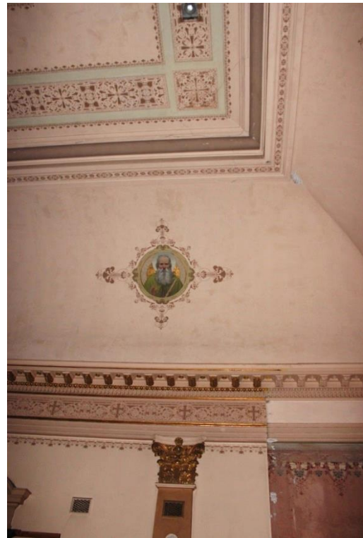
FIGURE 28. CHURCH: NAVE CEILING, DETAIL OF ORNAMENT ON COVED SECTION, 2016.
