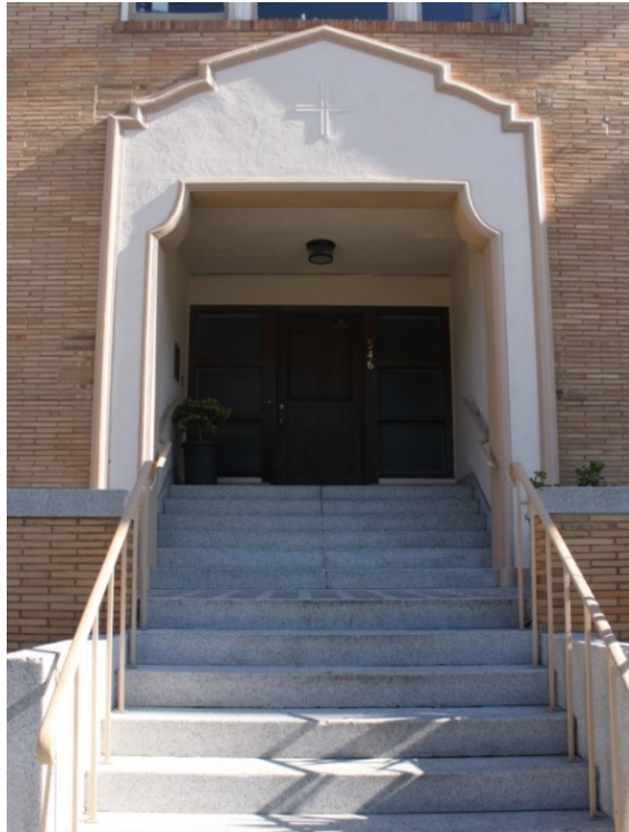
FIGURE 39 (LEFT). RECTORY: MAIN ENTRANCE, 2015.
