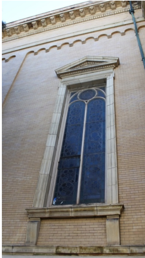
FIGURE 9. CHURCH: NORTH ELEVATION, DETAIL OF WINDOW, LOMBARDY BAND, AND CORNICE, 2015.
