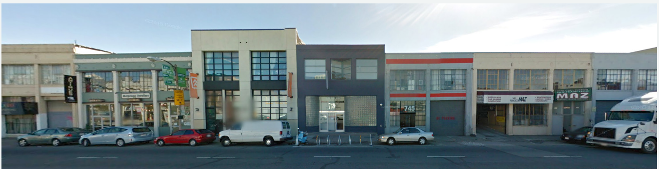
Bryant Street elevation. Photo by Google Maps
