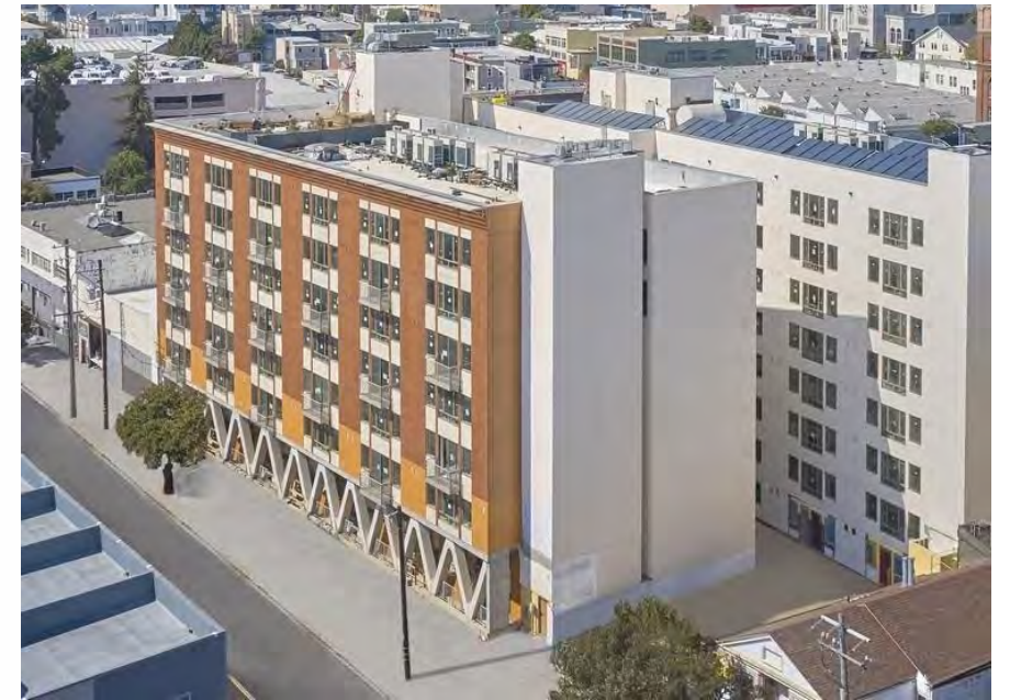
City Gardens – 200 Units of Supportive Housing for Families
