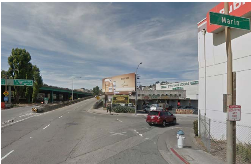
Figure 3: Segment M (Looking North at Marin St. and Bayshore Blvd.)
