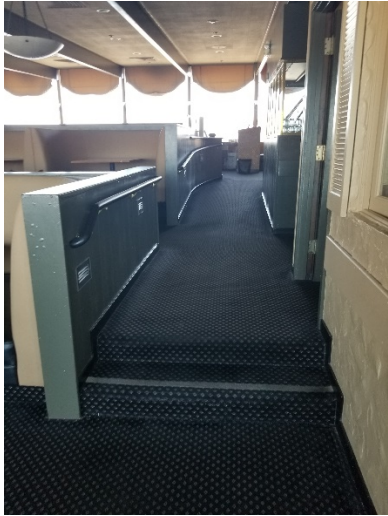
Figure 76: 3 rd Floor Steps to Mid Dining
