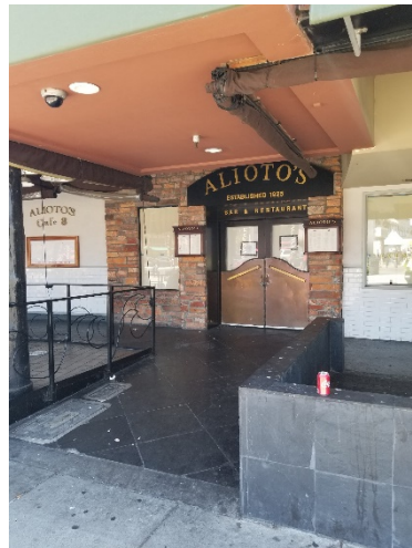
Figure 6: Entrance to Aliotos's Restaurant
