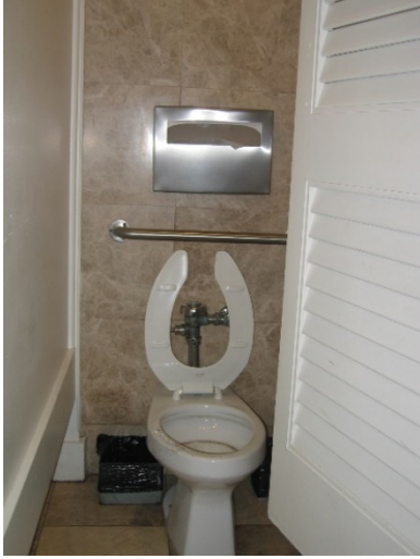
Figure 52: Figure 52: 2 nd Floor Women's Restroom
