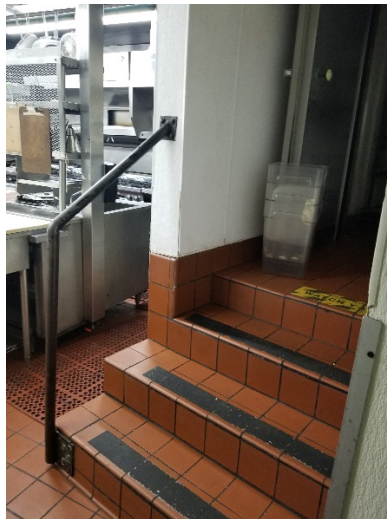
Figure 79: 3 rd floor Kitchen (Stair to Storage)
