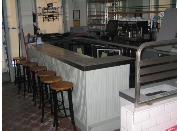
Figure 25: Side Door Entrance/Exit at Bar Counter
