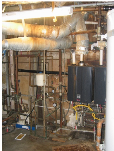
Figure 88: 2d Floor Mechanical Room
