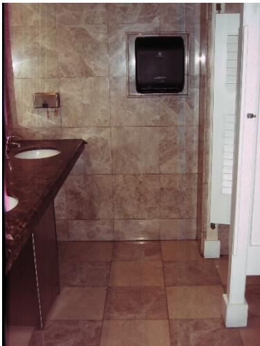
Figure 52: 2 nd Floor Women's Restroom
