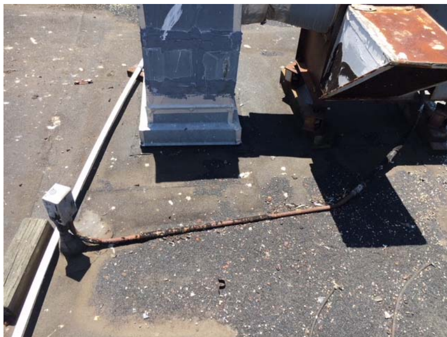
Figure 14 Unsupported conduit
