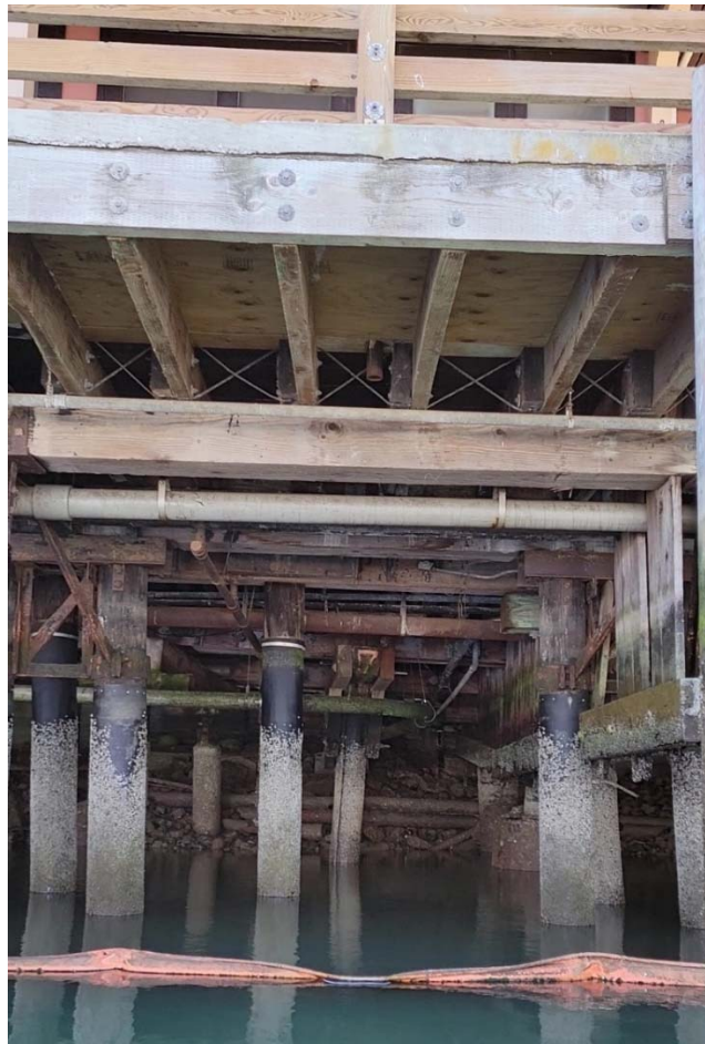
Figure 1 Photo of typical condition under Alioto's restaurant
