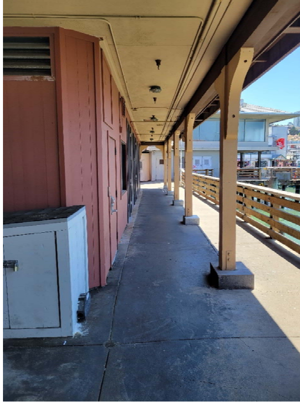
Figure 12 Ground Floor awning – west side
