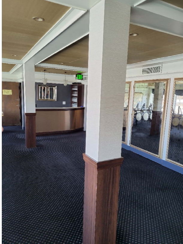
Figure 4 Column supporting third floor – Taken from 2 nd floor
