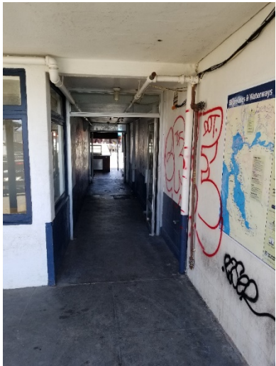
Figure 9: Door to Passage Way
