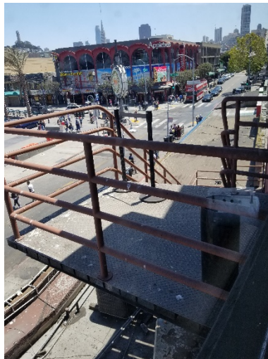
Figure 87: 3 rd Floor Exterior Egress Stair #4
