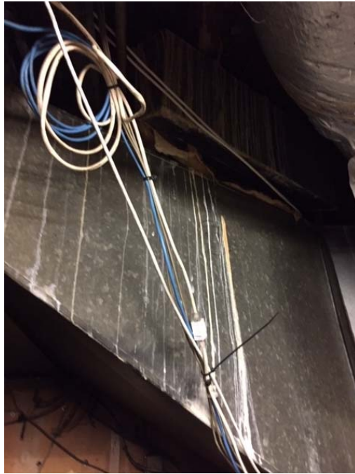
Figure 11 Employee Access Storage
