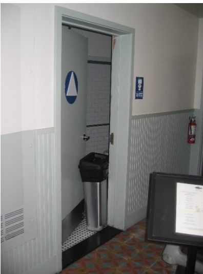
Figure 40: 1 st Floor All Gender ADA Restroom
