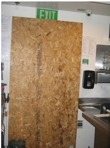
Figure 28: 1st Floor Bus Station
