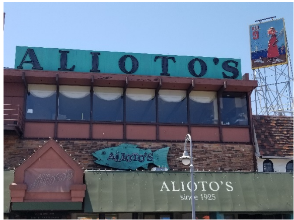
Figure 4: Closeup of Front Façade & Signage
