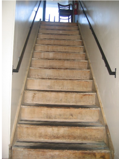
Figure 85: 3 rd Floor Rear Egress Staircase #3
