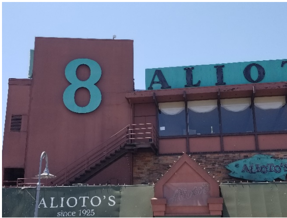
Figure 3: Closeup of Front Façade & Signage
