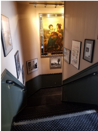
Figure 22: Staircase #1, missing Handrail Extensions
