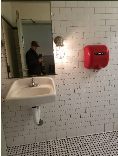
Figure 42: 1 st Floor All Gender ADA Restroom
