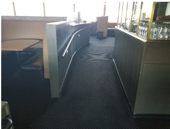
Figure 68: 3 rd Floor Ramp to Upper Dining Area
