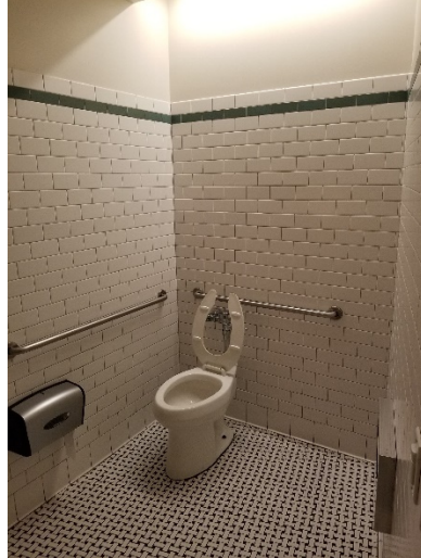
Figure 43: 1 st Floor All Gender ADA Restroom
