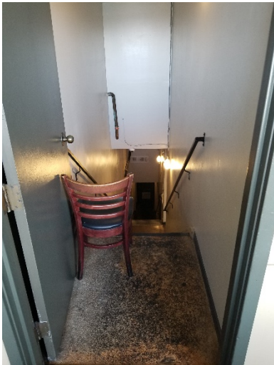
Figure 84: 3 rd Floor Rear Egress Staircase #3
