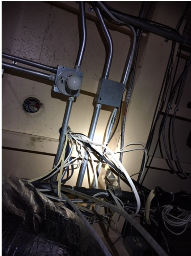
Figure 13 Romex 1st floor
