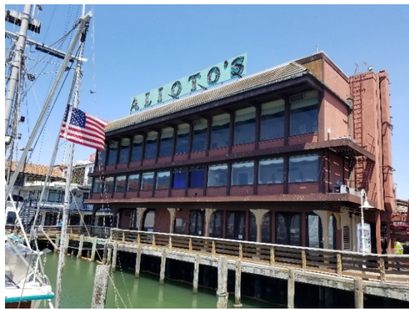
Figure 12: Rear of Alioto's/Wharf J-3
