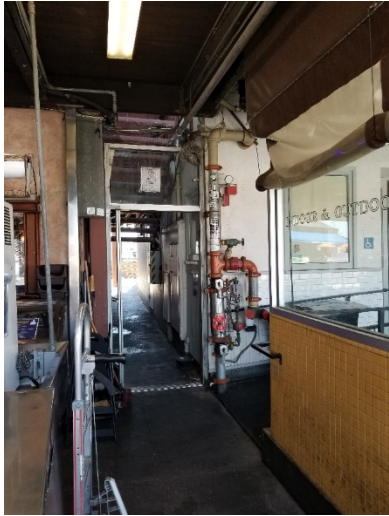
Figure 7: Door to Passage Way
