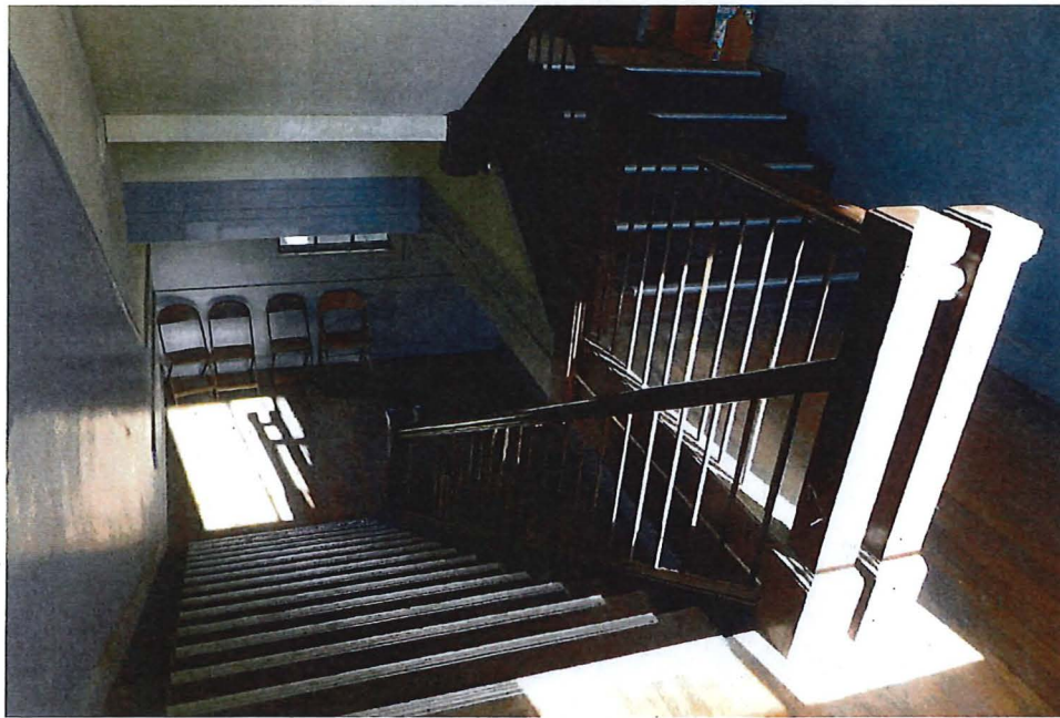
Dogleg, closed string wooden stairs with railing.
