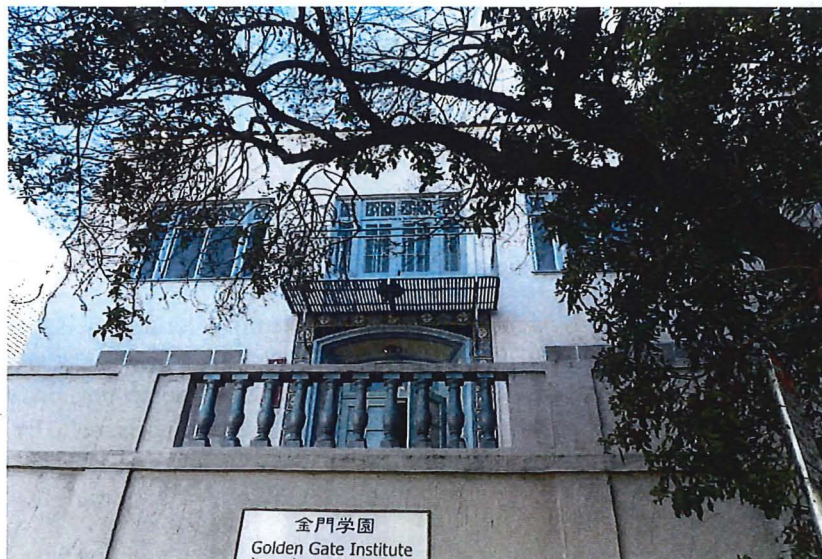
Primary (north) façade, view south.
