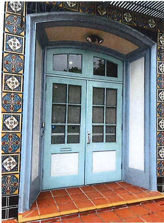
Main entrance, view southwest.
