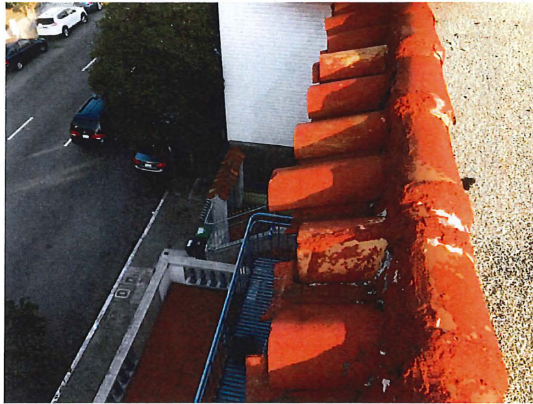
Detail of red clay tile coping at roof, view east.
