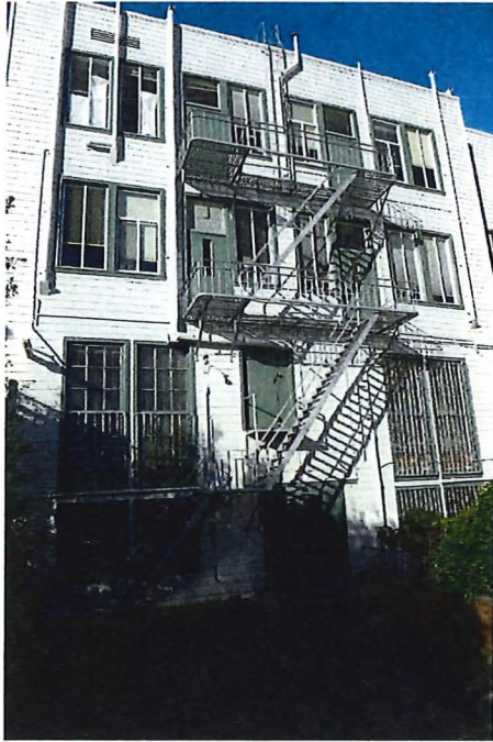
Rear (south) façade, view north.
