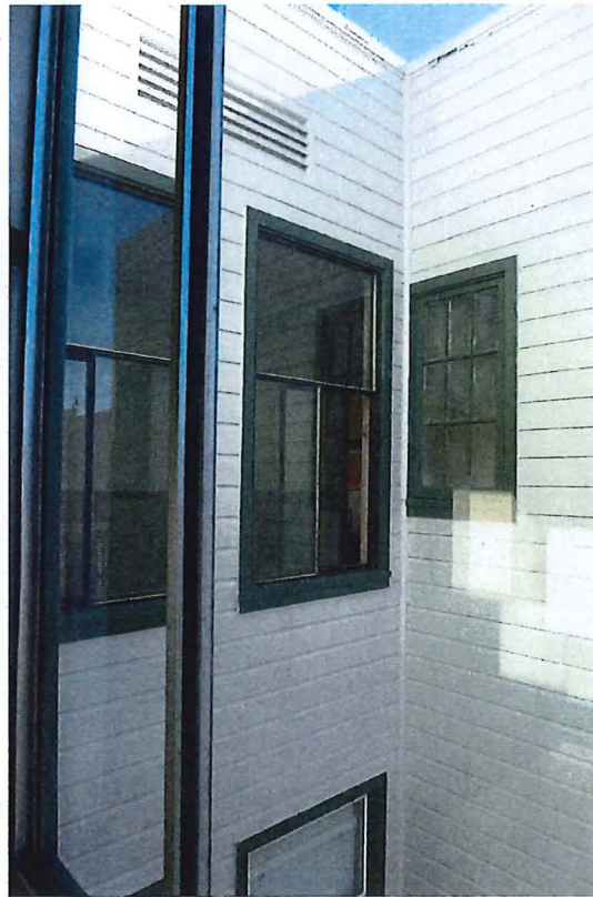
Light well at west elevation.
