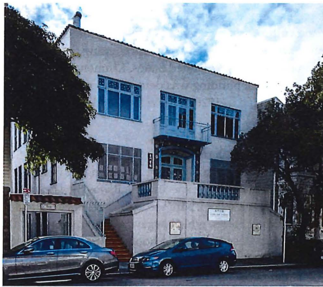
The Kinmon Gakuen Building, 2018.
