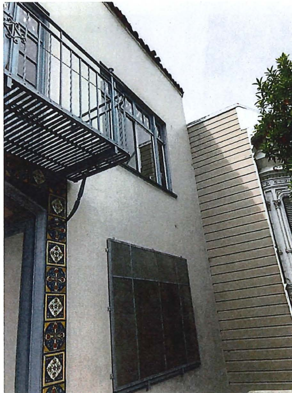
Detail at front façade, view southwest.
