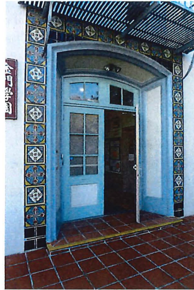
Detail of main entry at front (north) facade, view south.
