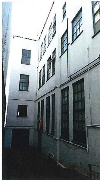
East elevation, view southeast.
