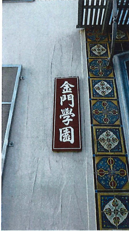
Japanese sign reading "Kinmon Gakuen" to left of main entry door, view south.
