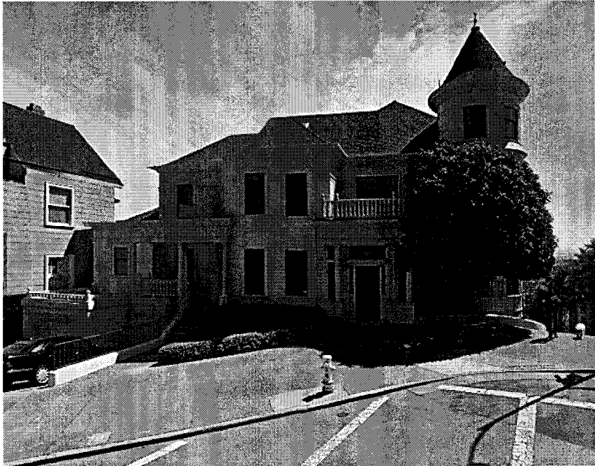
West façade of 181 Buena Vista East Ave. Image courtesy of Google, 2013.
