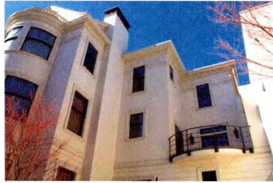
Figure 9. Upper stories of the third structural bay (rounded), fourth bay (recessed), and fifth bay (more recessed with balcony) on the east façade. Source: Page & Turnbull.
