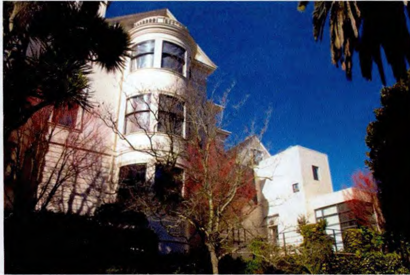
Figure 10. East façade, showing 1987 addition to the right (north). Source: Page & Turnbull.
