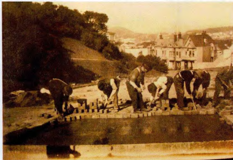
Figure 19: Paving on Buena Vista Avenue East, November 1916. Source: Department of Public Works Photo Archive, accessed at the San Francisco History Room at the San Francisco Public Library.
