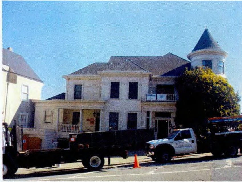
Figure 3: Primary (West) Façade, February 2013. Source: Page and Turnbull.
