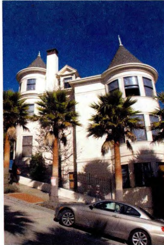
Figure 5: South Facade. Source: Page & Turnbull.
