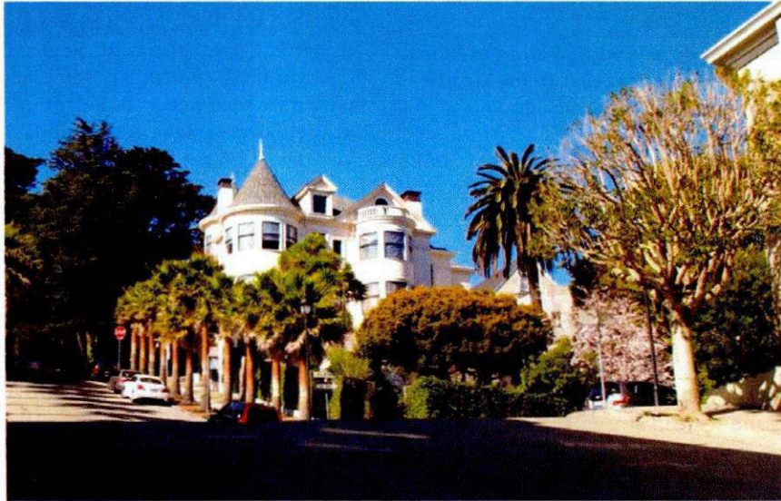
Figure 7. East façade, viewed from Duboce Avenue east of Alpine Terrace, showing dormers. Source: Page & Turnbull.
