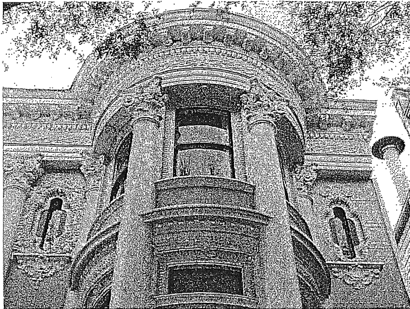
Figure 12: Bay flanked by oval windows in elongated quatrefoil surrounds (south window has a simpler surround).
