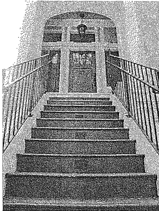
Figure 6: Exterior stairs leading to second story.
