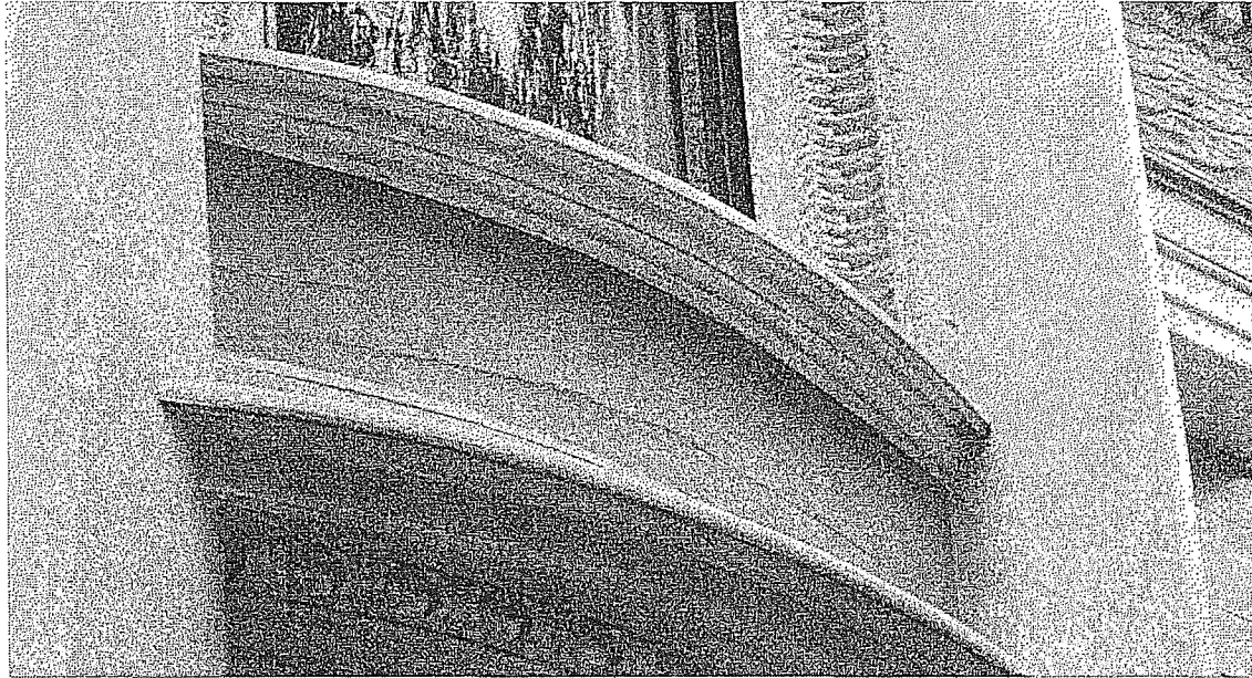
Figure 26: Detail of split wood panel between windows.
