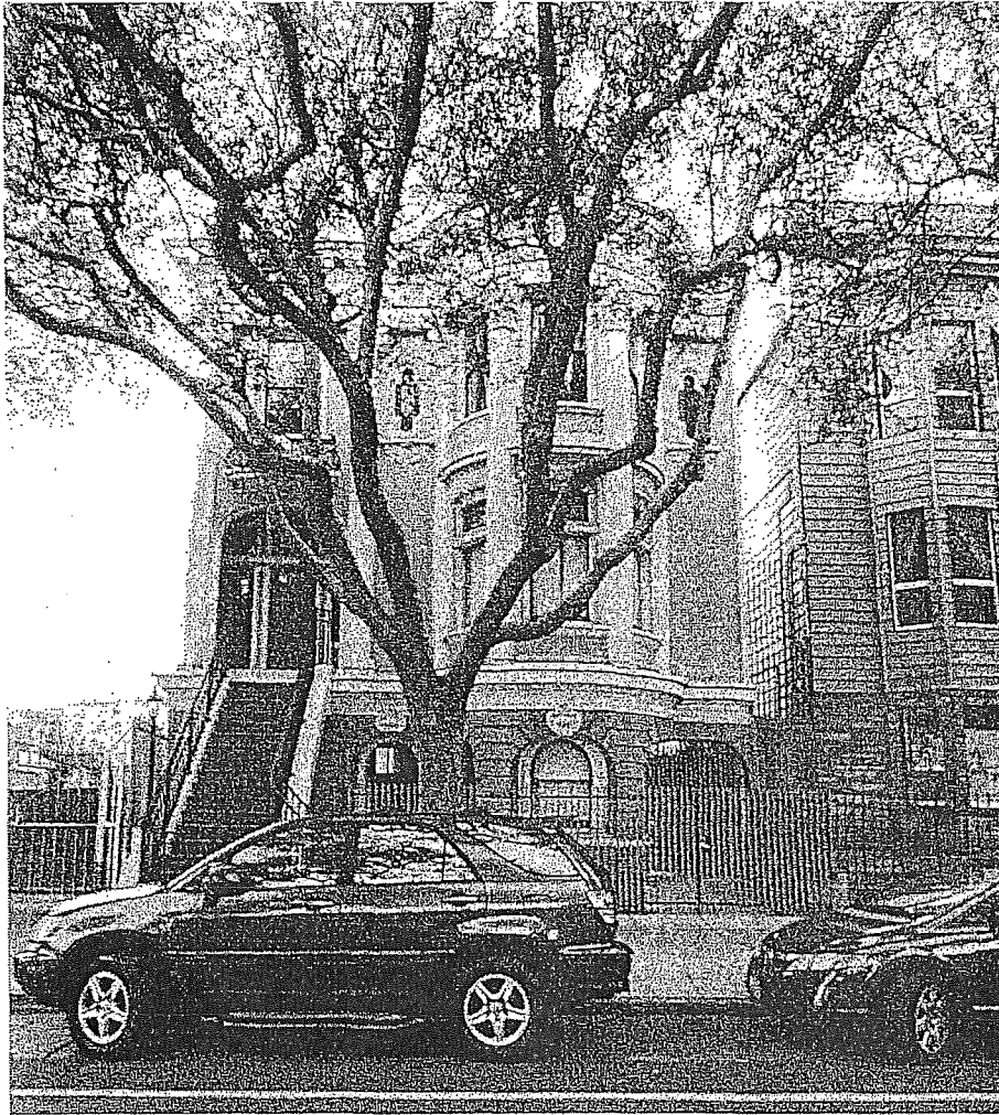
Figure 2: 2731-35 Folsom Street, primary facade, April 2017. Looking south.
