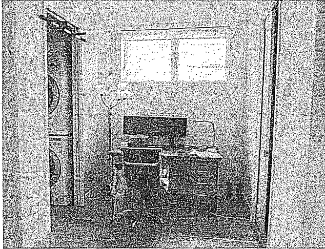
Photo 38: Level 1, office alcove Looking north
