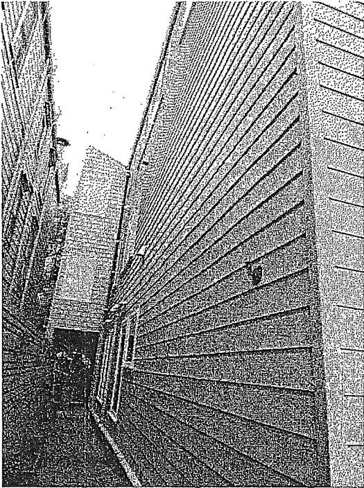
Photo 5: Side facade Looking west
