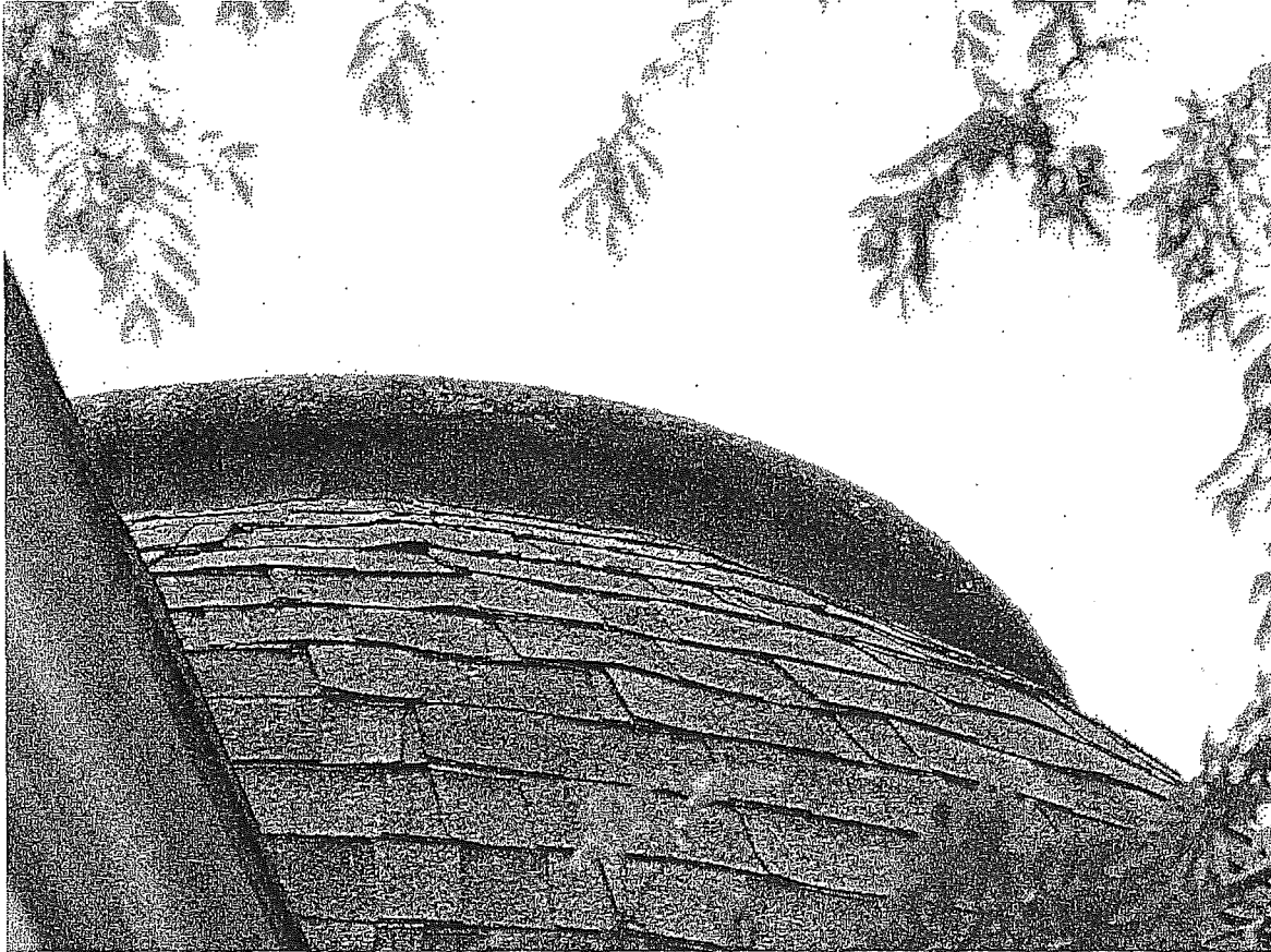
Figure 31: Detail of shingles at turret.
