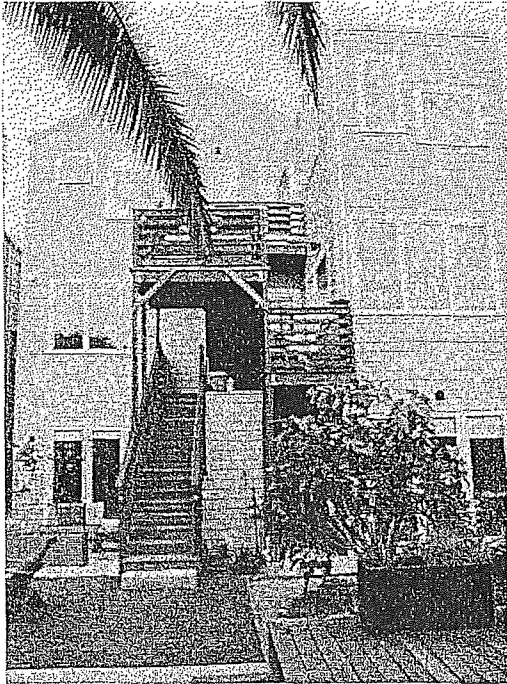
Figure 17: Rear (east) façade with south (left) and north (right) sides.
