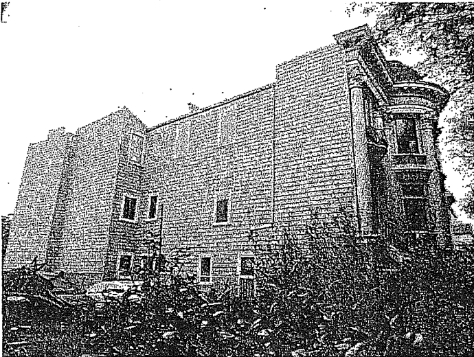
Photo 3: Side facade Looking south
