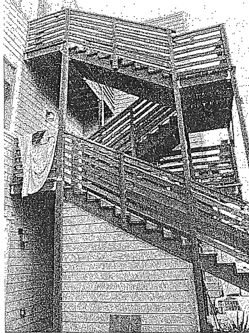
Figure 18: Exterior three-story stairs.
