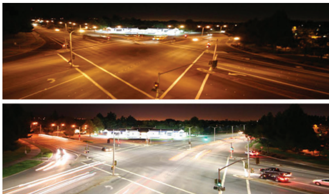
Figure 4. Before (top) and After (bottom): All Fremont streetlights were fully converted to brighter LED lights (16,000 lights).
