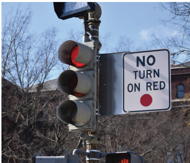
Figure 2. No Turn on Red Installation at 15th Street and Independence Avenue, SW.
