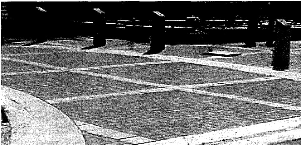
Permeable pavement can be integrated into a variety of hardscapes such as roads and sidewalks, plazas, terraces and patios.
