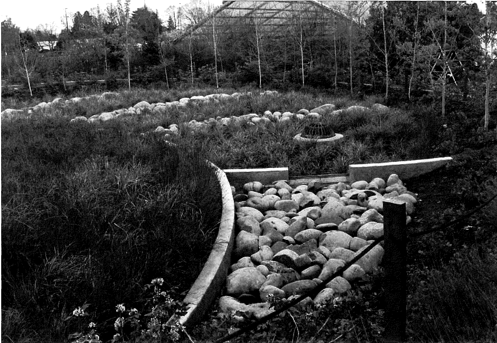
A rain garden at Glencoe Elementary in Portland, Oregon reduces stormwater flows to Portland's collection system.
