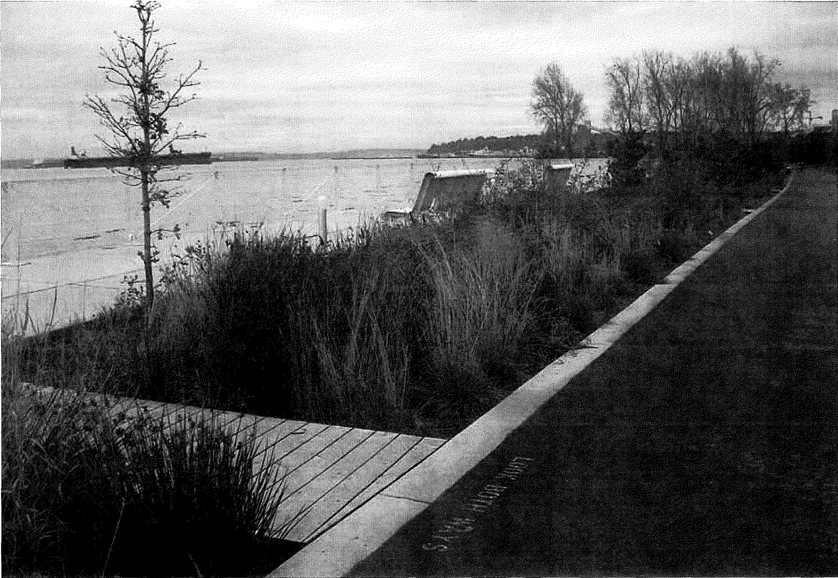
Boardwalks provide access across waterfront bioretention facilities in Seattle, WA.
