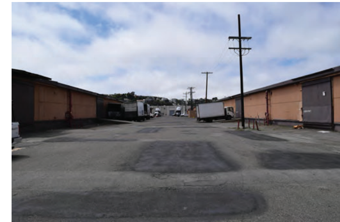
12 FROM SELBY ST, W THROUGH SITE
