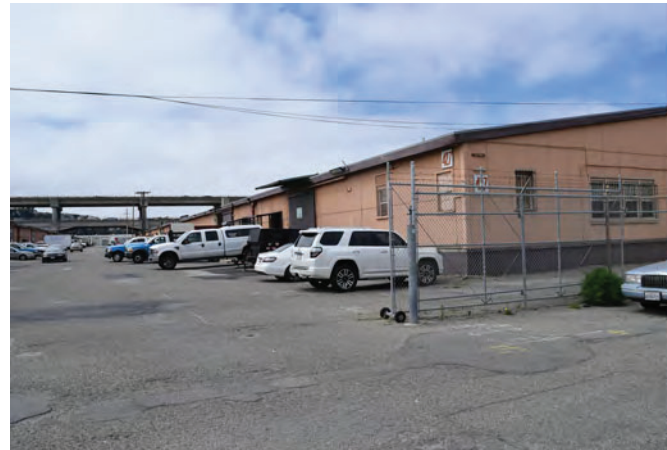
11 FROM RANKIN ST, SITE ENTRANCE
