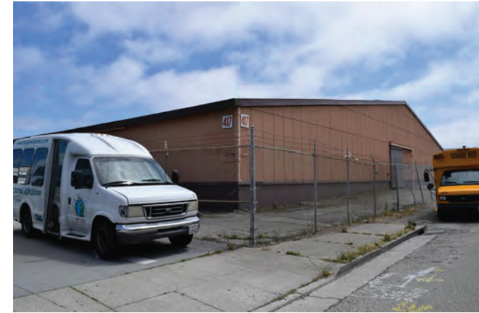
9 FROM TOLAND ST, NW CORNER OF SITE
