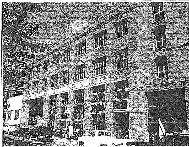
Garcia and Maggini Warehouse, 128 King Street
