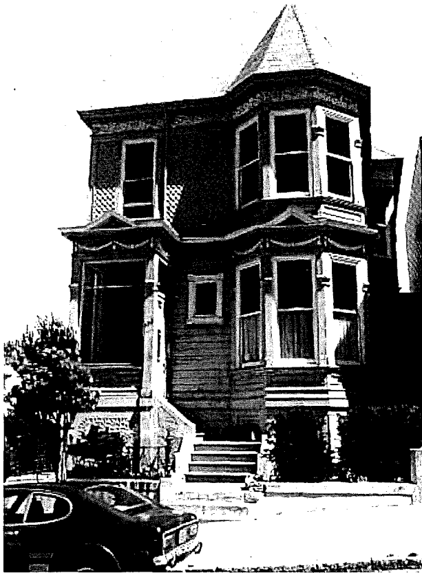
Figure 5. 722 Steiner Street, ca. 1976. In this photo, the portico has been closed in, and the exterior appears similar to how it looks today. The gate spanning the walkway to the south appears to be constructed of horizontal wood siding. (Photograph from San Francisco Planning Department, April 2015.)
