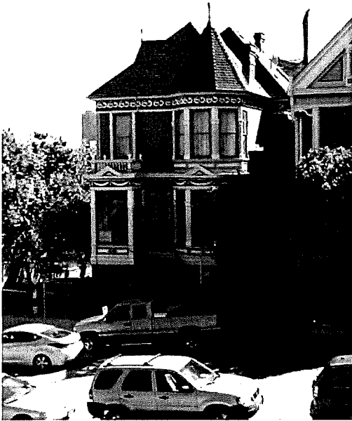
Figure 8. Overall view of west (Steiner Street) elevation. (Photograph by Garavaglia Architecture, Inc., April 2015.)
