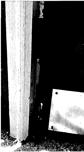
Figure 24. Rotted wood at entrance portico door. (Photograph provided by Côme Lague, April 2015.)
