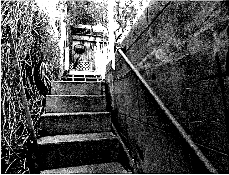
Figure 17. Detail of handrail. (Photograph provided by Côme Lague, April 2015.)
