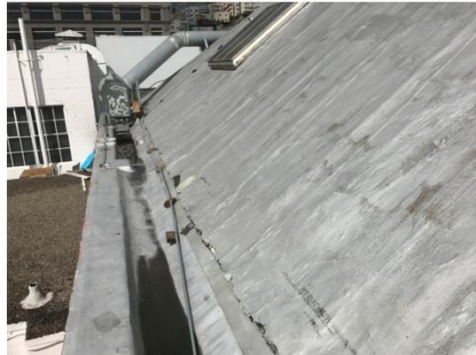
Photo 4: Steep slope roof with aluminum roofing coating.
