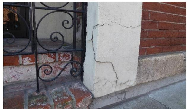
Figure 21 Detail photograph of cracked and spalling cement plaster (photography taken on 03/31/2017).
