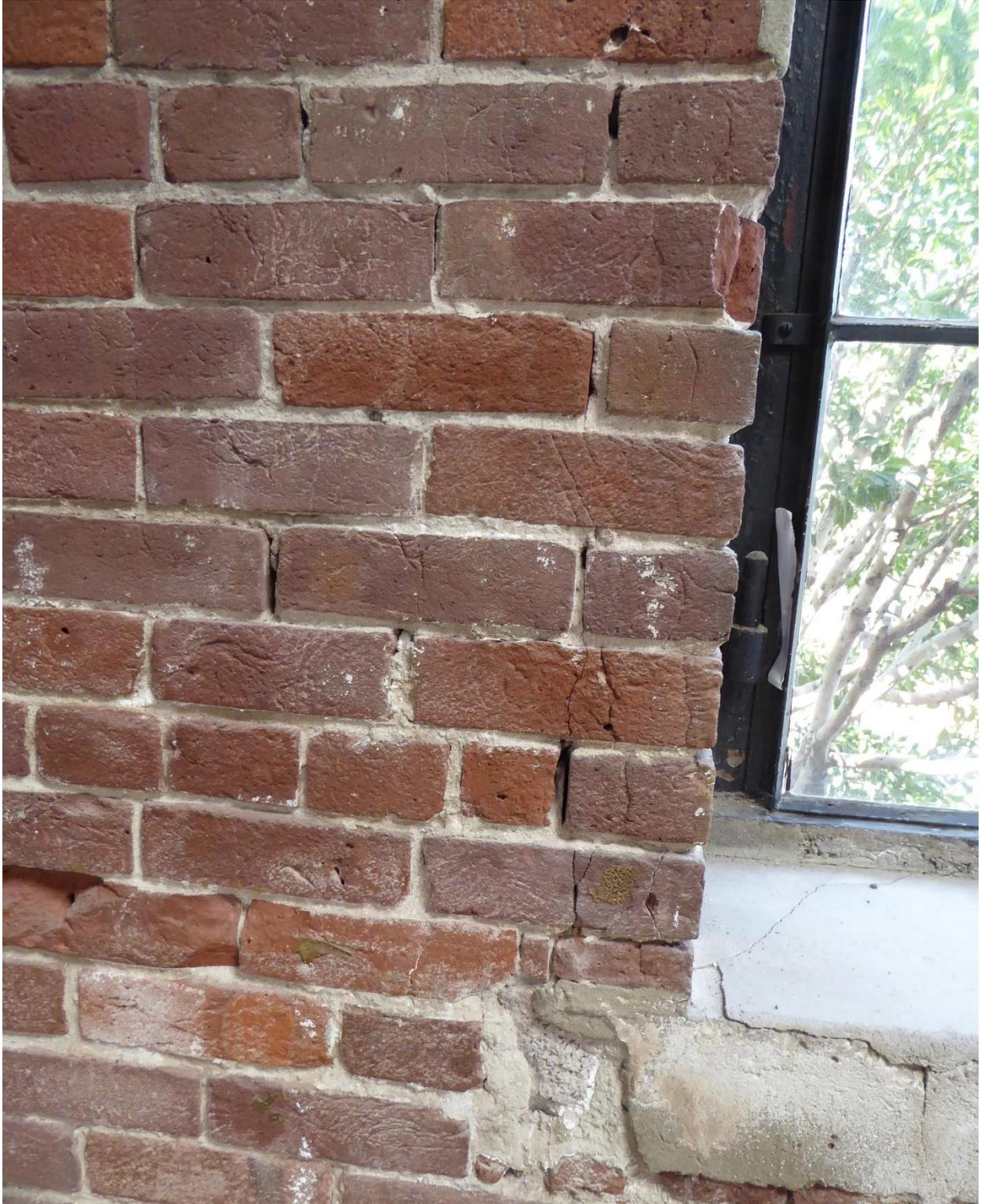
*Figure 133 Typical condition of cracked bricks around window openings (photograph taken on 04/10/2017).*
