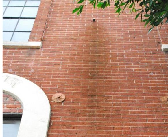
Figure 35 Non-functioning downspout along Vallejo Street. The inability to direct water away from the facade and foundation have resulted in heavy areas of bio-colonization. This will, in turn, accelerate the deterioration of the brick and mortar (photography taken on 03/31/2017).
