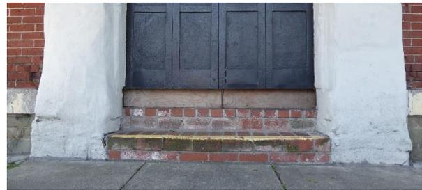
Figure 9 Detail view of entryway. Note brick stairs and biological growth (photography taken on 03/30/2017).
