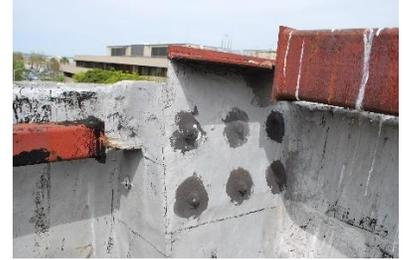
Figure 42 Detail of extant hollow-steel-beam, bolt plate, and concrete pier construction (photography taken on 04/05/2017).
