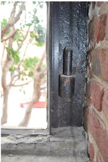
Figure 128 Detail photograph of window hardware on the second floor. Four of these are used in each window, two lower and two upper. This is believed to be the earliest construction type found for the windows (photograph taken on 04/04/2017).
