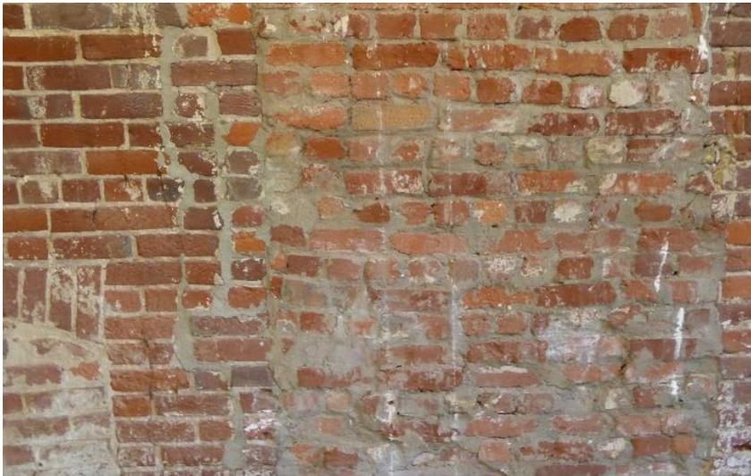
Figure 65 Detail photograph of historic window filled-in with brick on the east wall. There are 4 similar conditions on this elevation (photography taken on 04/10/2017).
