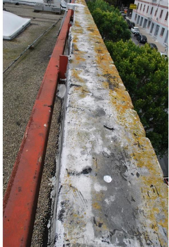
Figure 52 Photograph of horizontal surface on east parapet. Note biological-colonization, corrosion, atmospheric soiling, and minor animal deposits (photography taken on 04/04/2017).
