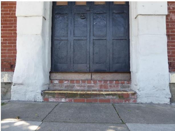
Figure 89 Detail view of entrance bay along Front Street. Note biological activity on brick coursework (photograph taken on 03/30/2017).
