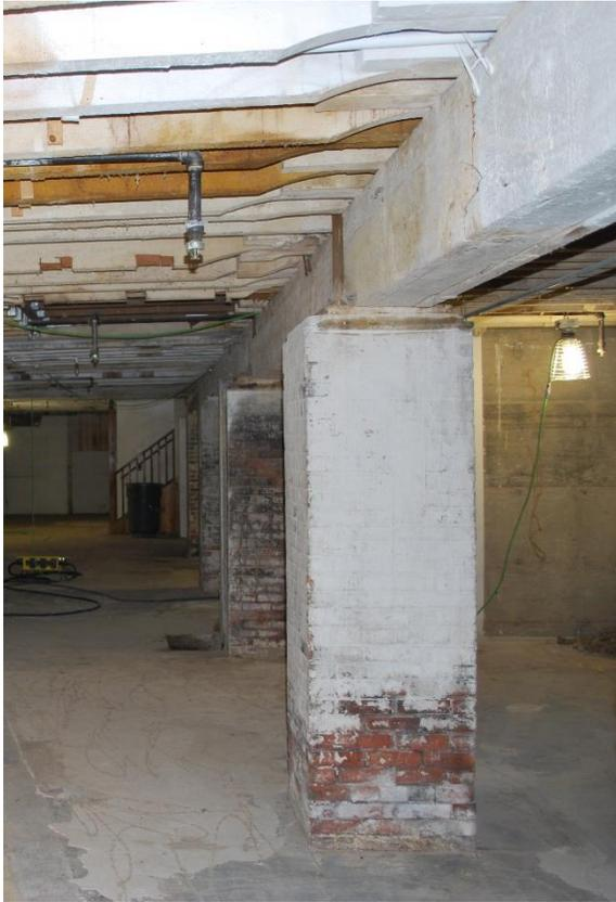
Figure 71 Photograph of structural timber beam to brick pilaster connection (photography taken on 04/04/2017).
