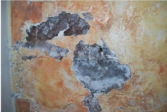
Figure 75 Detail photograph of north foundation condition. Note lost finish, exposed stone, and extensive efflorescence (photography taken on 04/04/2017).
