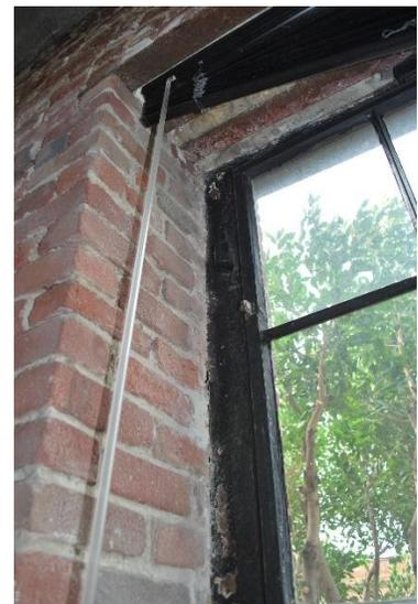
Figure 130 Detail photograph of window hardware on the second floor. Same window as previous two images. This is believed to be the earliest construction type found for the windows (photograph taken on 04/04/2017).
