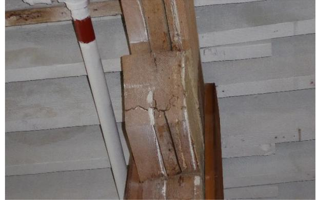
Figure 108 Interior detail of structural timber construction. Note split in capital (photograph taken on 04/10/2017).
