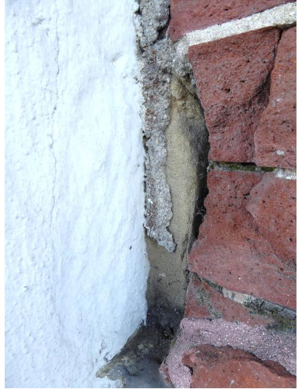
Figure 92 Photograph of entrance threshold at Front Street elevation. Note sandstone substrate (photograph taken on 03/31/2017).
