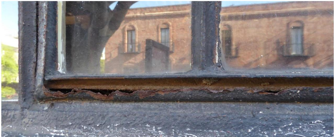
Figure 26 Detail of localized corrosion and window sash failure. Instances are few, however, need repair/rehabilitation (photography taken on 03/31/2017).
