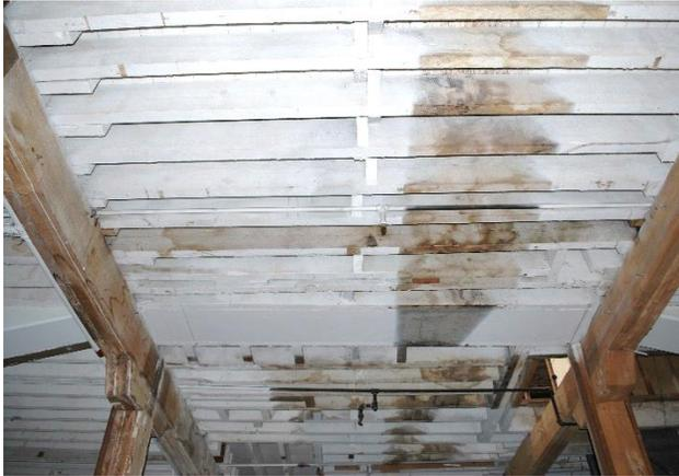
Figure 103 Photograph of ground floor ceiling joists. Note ghosts from old HVAC and water staining (photograph taken on 04/04/2017).
