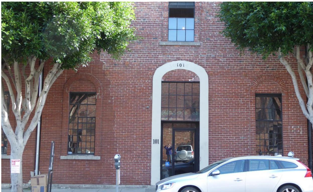
Figure 27 Photograph of 101 Vallejo Street. Note visual seam between historic brick (left) and the brick used in a later restoration campaign (right). Photography was taken on 03/30/2017.
