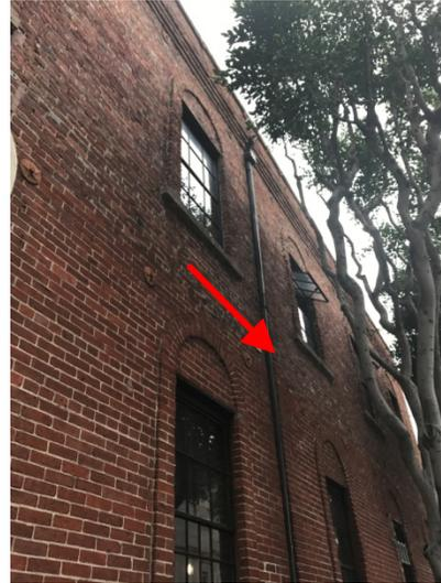
Photo 22: Downspout from through-wall drain.
