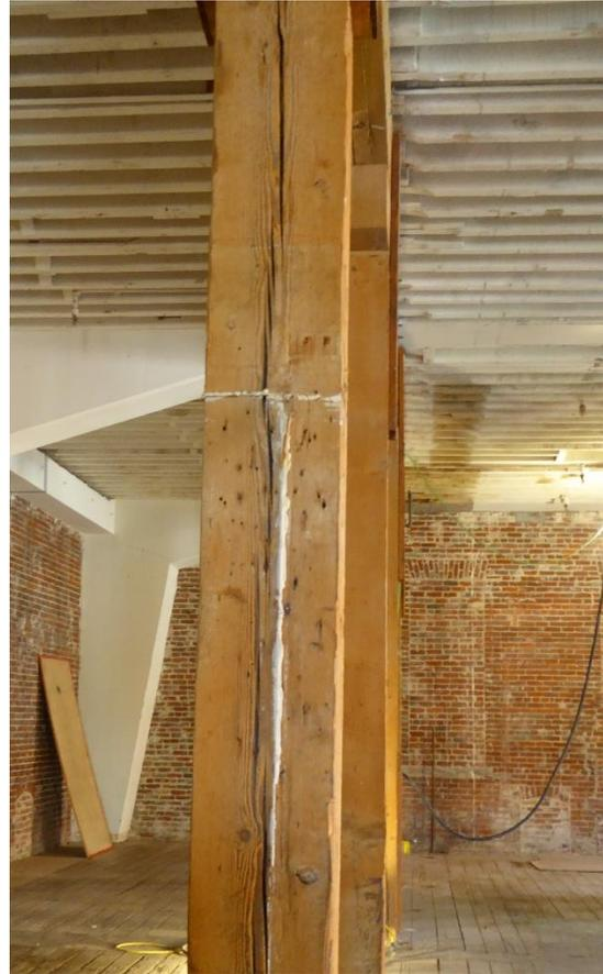
Figure 59 Interior photograph of vertical splitting present in several of the structural timber columns on the ground floor (photography taken on 04/05/2017).
