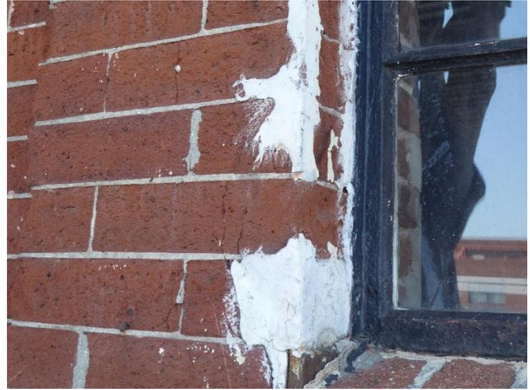
Figure 14 Detail of inappropriate repair material used on the brick façade (photography taken on 03/30/2017).
