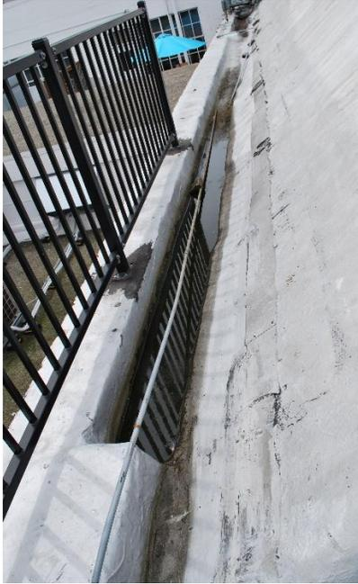
Figure 39 Detail photo of drainage condition along the south parapet. Note standing water (photography taken on 04/05/2017).
