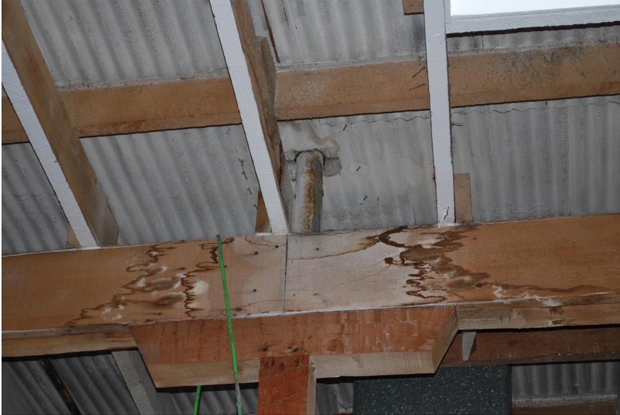
Figure 82 Detail of roof to beam construction. Note water staining and efflorescence on wooden members (photography taken on 04/04/2017).
