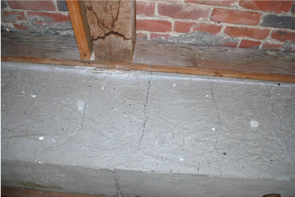
Figure 80 Detail of modern lateral stabilization system (concrete beams). Note severe through-cracking of the cement matrix (photography taken on 04/04/2017).
