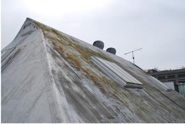
Figure 45 Detail of north facing hip of the roof. Note heavy biological colonization (photography taken on 04/05/2017).
