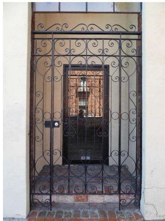
Figure 97 Detail photography of easternmost entrance along Vallejo Street. Note stucco over brick threshold, metal security gate, and modern aluminum frame door (photograph taken on 03/30/2017).
