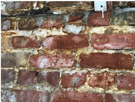
Photo 9: Deterioration in mortar joints of brick wall below gutter.
