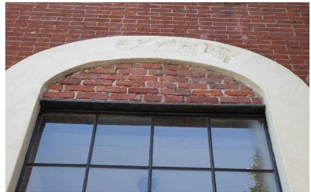
Figure 20 Detail of blind arch at westernmost entrance along Vallejo Street. Note the loss of concrete plaster and the raised metal rebar. Condition is also observed at the 101 Vallejo entrance (photography taken on 03/30/2017).
