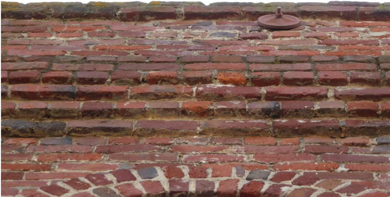
Figure 98 Detail view of corbeled cornice and parapet wall along Vallejo Street (photograph taken on 03/30/2017).
