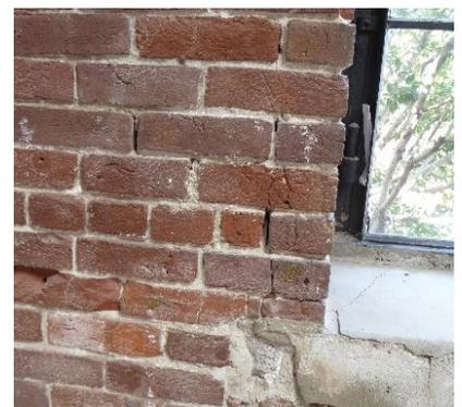
Figure 86 Detail of typical brick condition for deteriorated bricks around window openings (photography taken on 04/04/2017).
