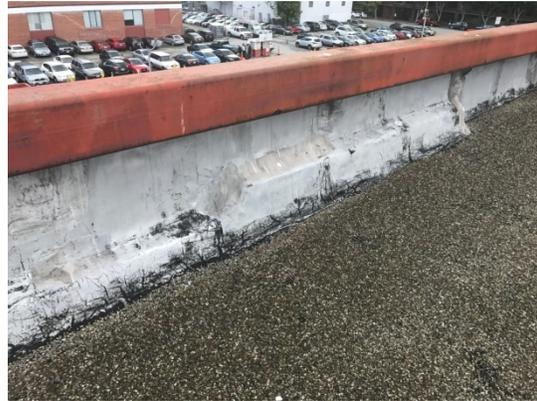
Photo 18: Roof sheet extends up brick parapet.
