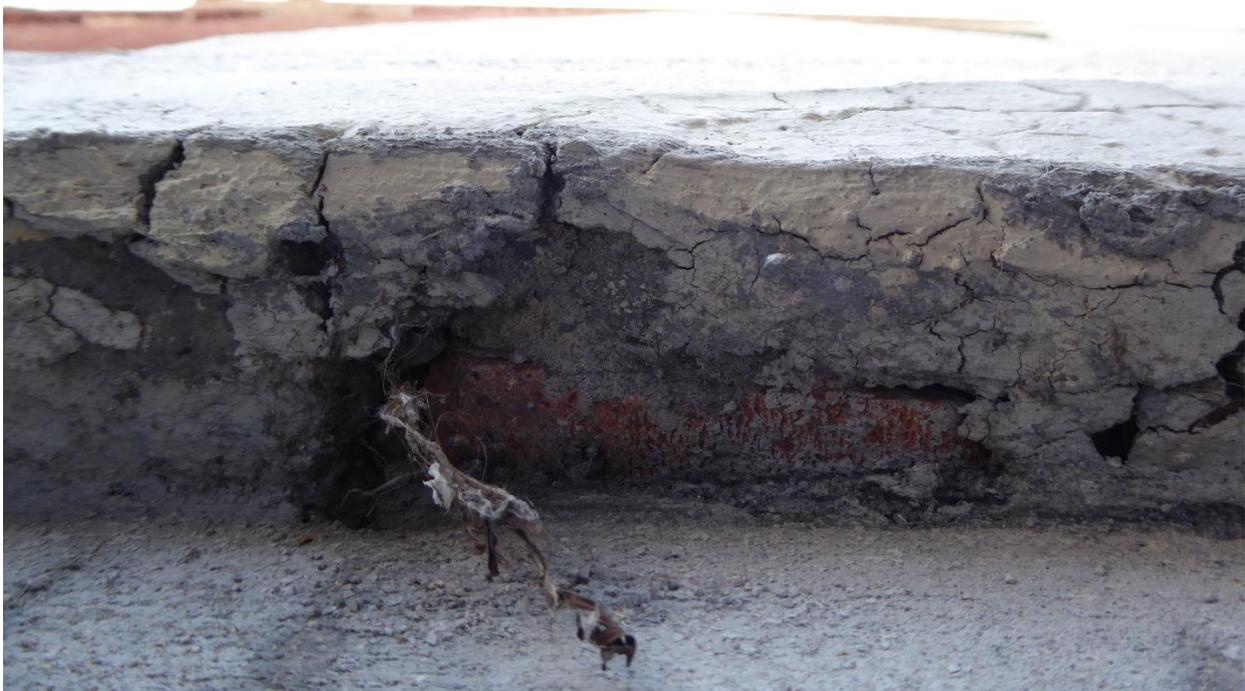
Figure 99 Detail view of cement stucco over brick construction along the Vallejo Street entrances (western two entrances). Photo taken from the foundation and looking up towards the cornice (photograph taken on 03/30/2017).
