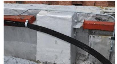
Figure 43 Detail of extant hollow-steel-column to concrete pier construction (photography taken on 04/05/2017).
