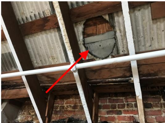
Photo 5: Hole from underside of steep slope roof that shows the variety of layers.
