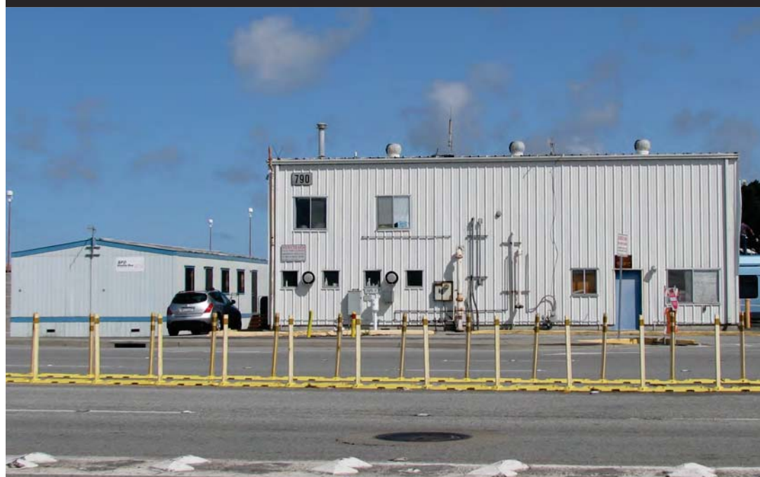
PHOTO 2: SFO SHUTTLE BUS - OFFICE TRAILER (LOOKING NORTH)
