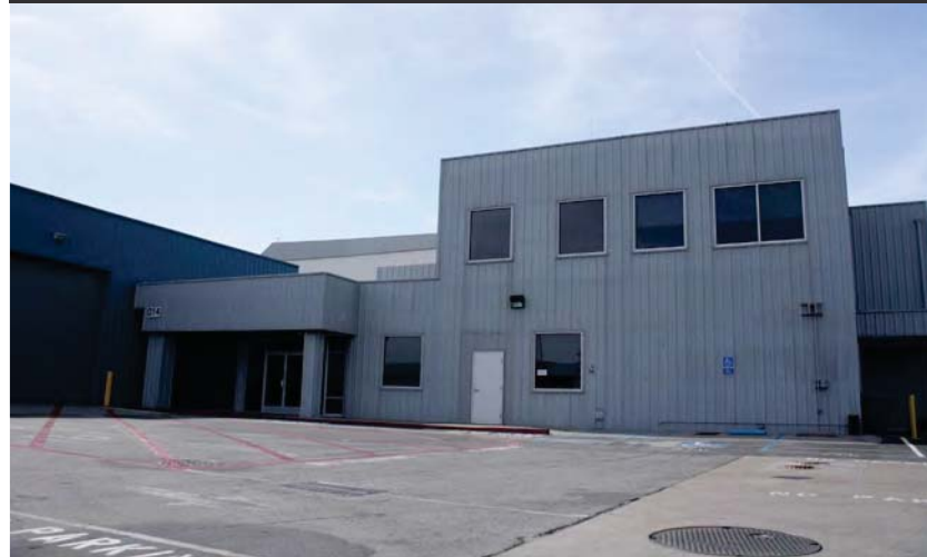
PHOTO 2: SFO GTU GARAGE (LOOKING NORTHEAST)
