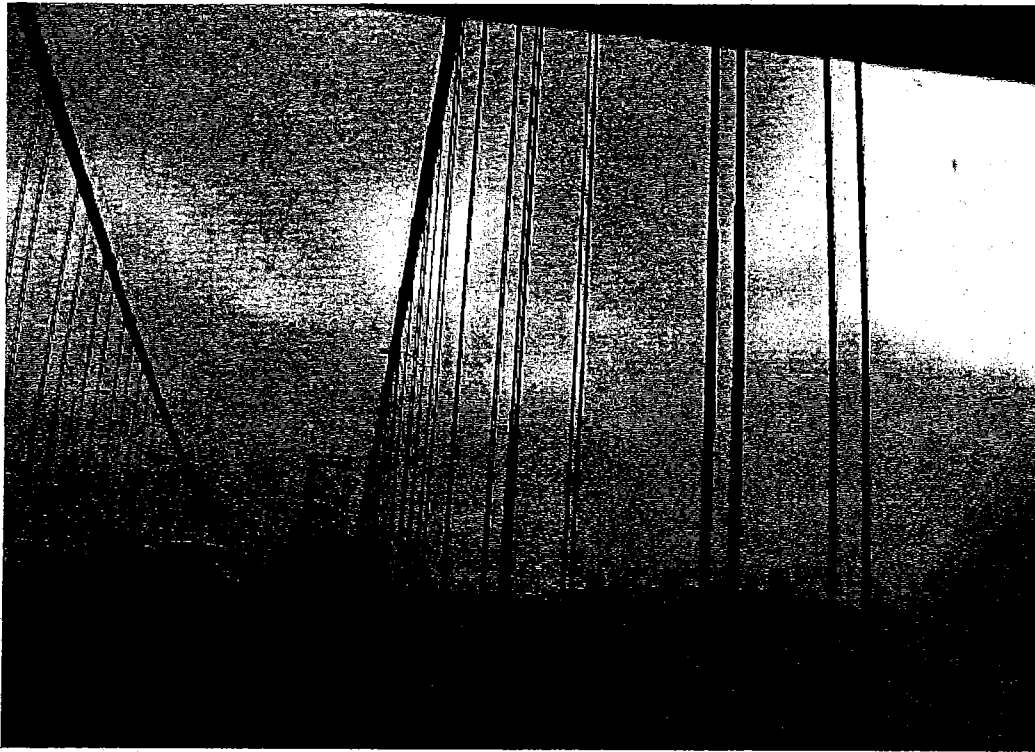
Photo 15: View of suspender cables of Bay Bridge looking west, toward the San Francisco shoreline, from Bay Bridge.
