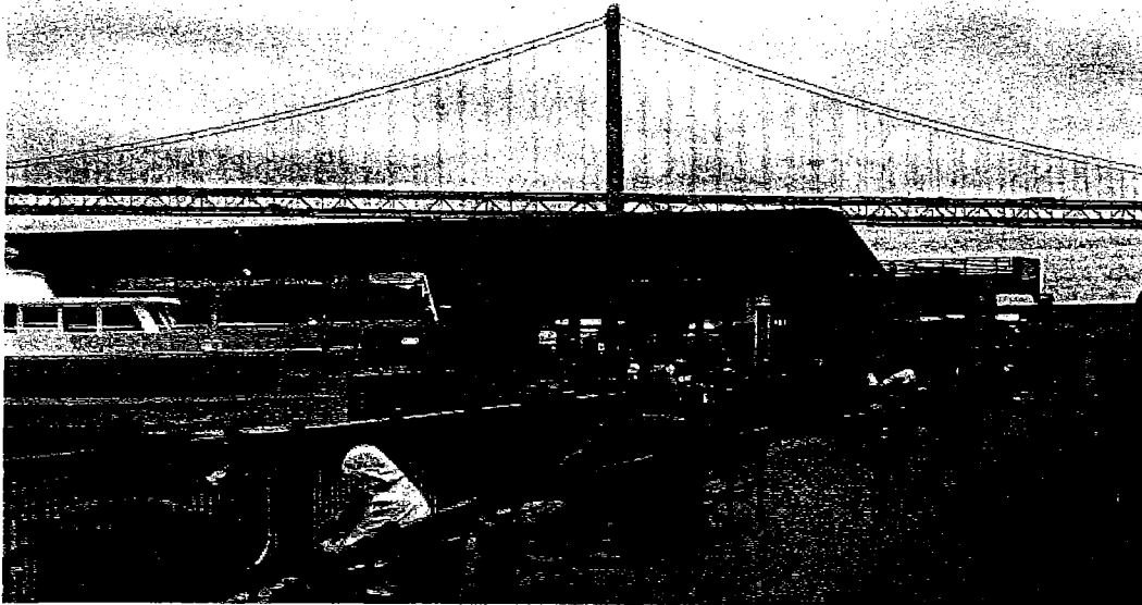
Photo 11: View of Bay Bridge looking east from the San Francisco shoreline from Ferry Building.
