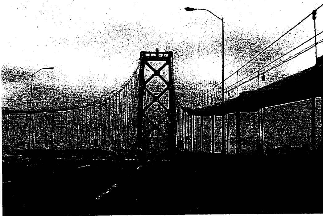
Photo 14: View of tower and suspender cables of Bay Bridge looking west, toward the San Francisco shoreline, from Yerba Buena Island on-ramp.
