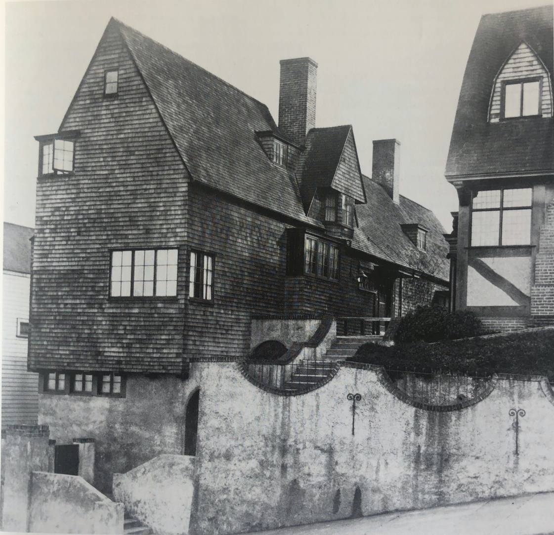
COXHEAD, Coxhead house (early photo), San Francisco, 1893
