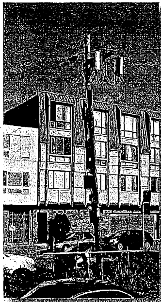
Crown Castle, for Verizon Wireless "oDAS XL" Personal Wireless Services Facilities, in the Outer Sunset. The bulky nature and potential noise generation from cooling fans on residential streets is disfavored.
