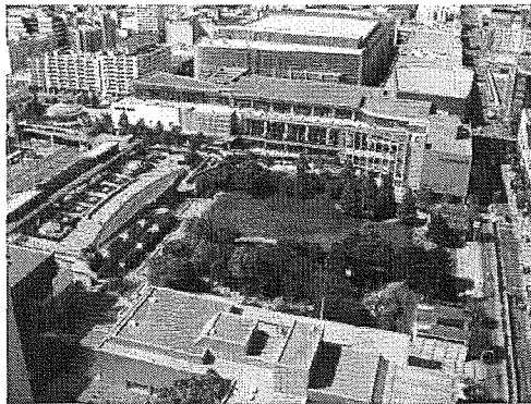
Aerial of Yerba Buena Gardens Open Space
