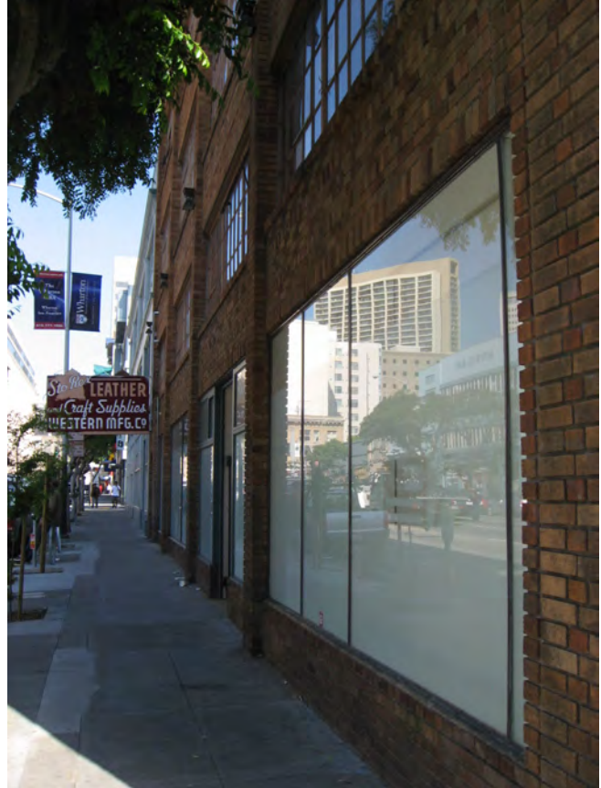
Figure 1. Typical Storefront at west elevation.
