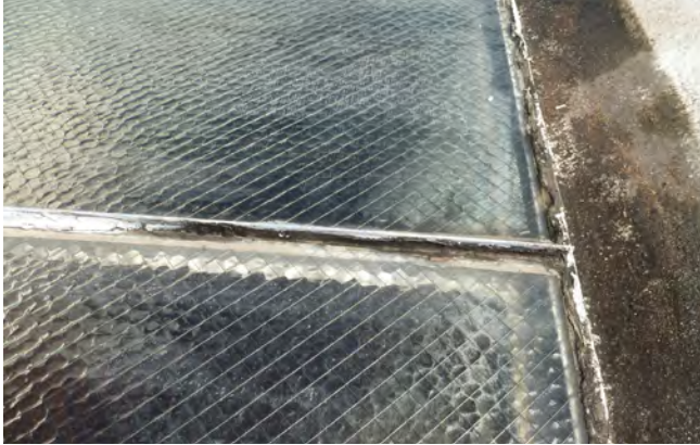
Figure 3. Skylight typical frame conditions.
