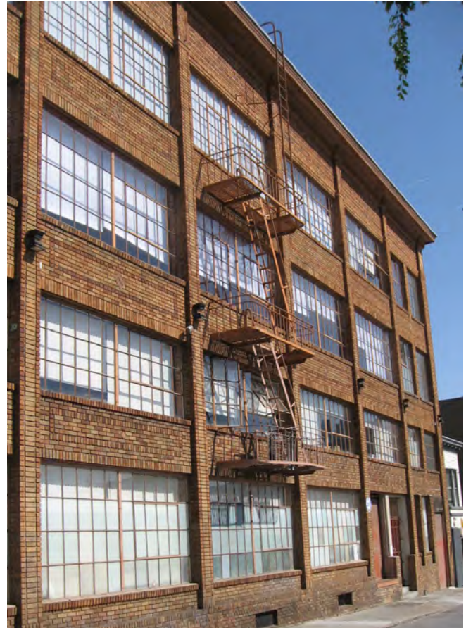
Figure 1. Metal fire escape at south elevation.
