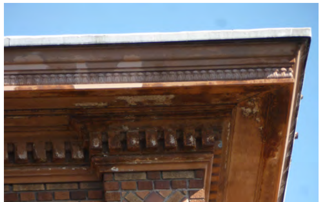
Figure 5. Cornice at southwest corner.
