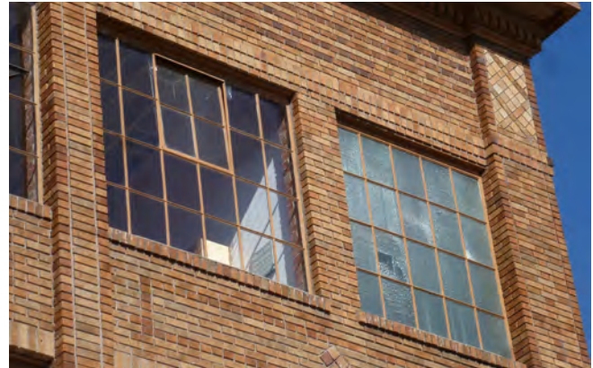
Figure 1. Typical multi-lite steel windows; note operable sections and glazing types.
