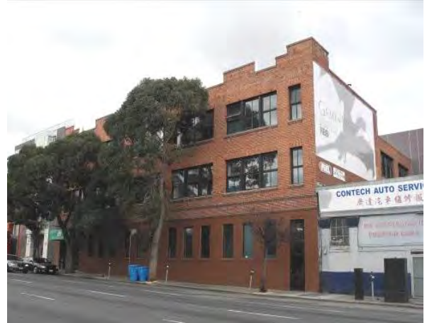
291 10 th Street, E.W. Bennett and Co. Building (1909). (Page & Turnbull, October 2013)
