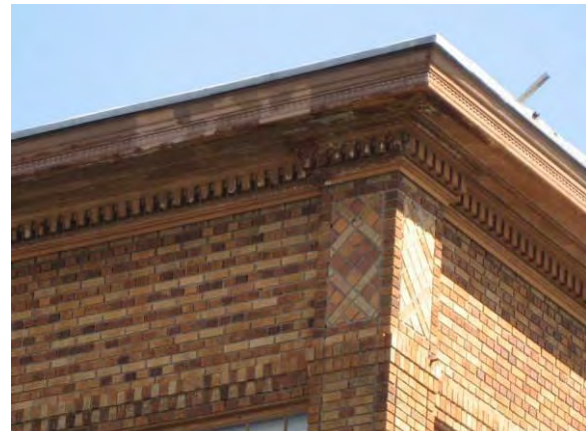
View of entries on the south façade (top) and detail of cornice at the southwest corner. (Page & Turnbull, April 2013)
