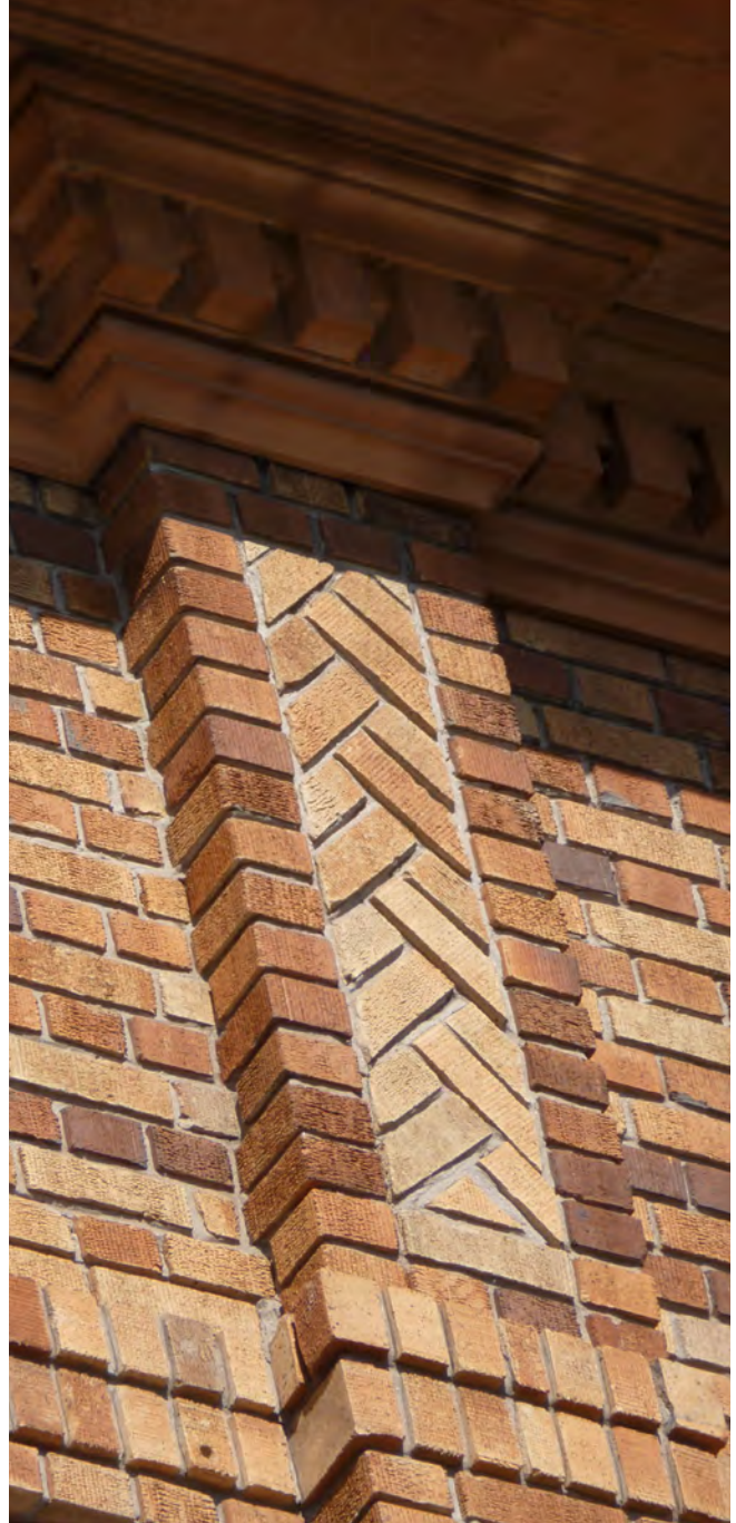
Figure 4. Detail of decorative brickwork at piers.
