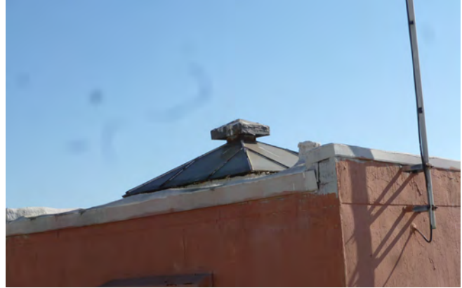
Figure 1. Roof & ventilator at penthouse.
