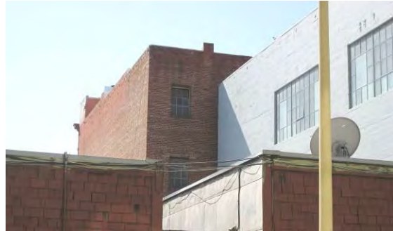
View south from Minna Street showing exposed portion of the north façade. (Page & Turnbull, April 2013)
