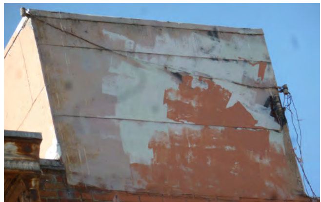
Figure 2. Penthouse from grade (east elevation).
