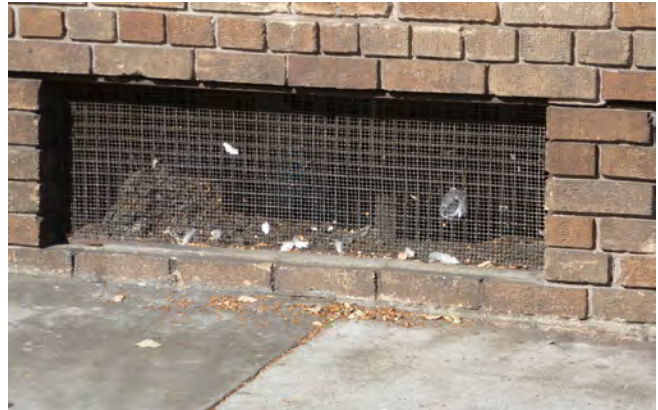
Figure 1. Ventilation grilles; note 1'x1' historic iron grille.
