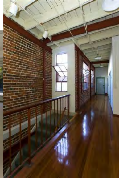
Third floor stair landing and windows on north wall.
