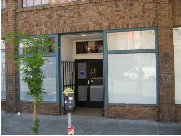
Detail of entry for 155 9 th Street. (Page & Turnbull, April 2013)
