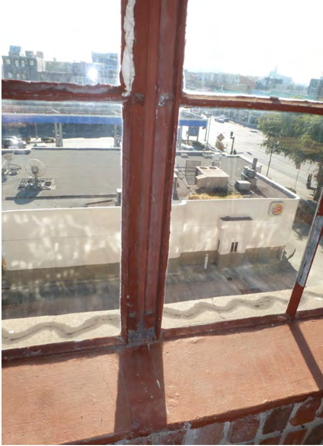
Figure 3. Steel window frame detail.
