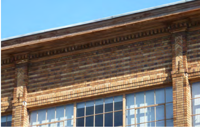
Figure 2. South Elevation; note dentils and decorative piers.
