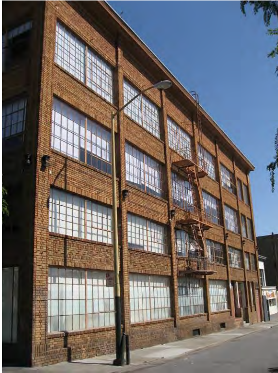
South façade of the building looking east. (Page & Turnbull, April 2013)
