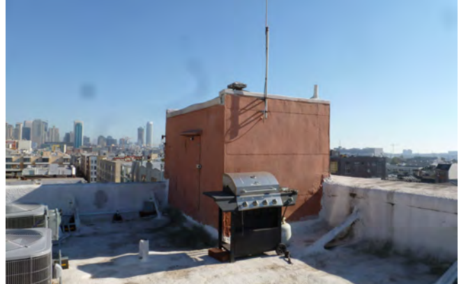
Figure 1. Penthouse from roof, typical.
