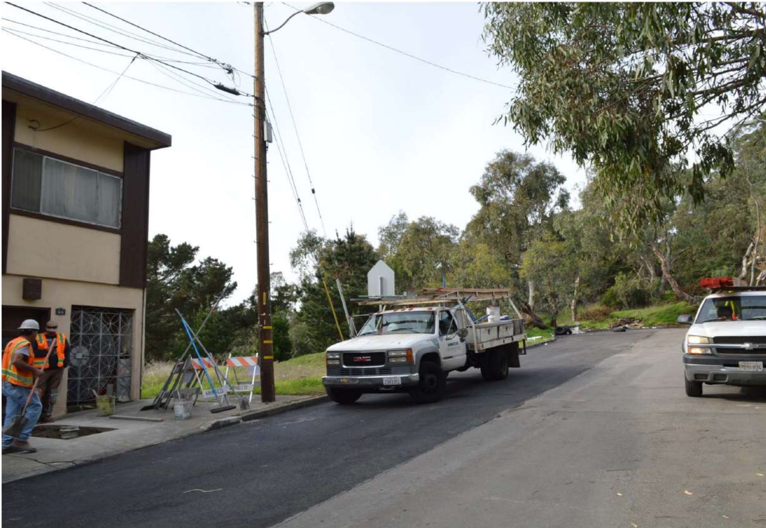
View #3 Raymond Avenue looking west
