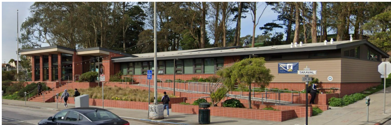
Parkside Branch Library, front façade, view northwest, 2023. Source: Google Streetview
