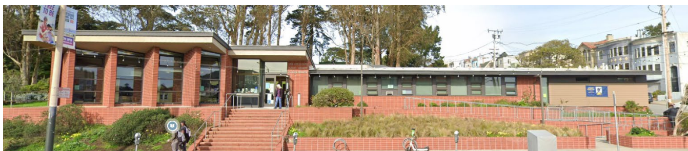
Parkside Branch Library, front façade, view north, 2023. Source: Google Streetview
