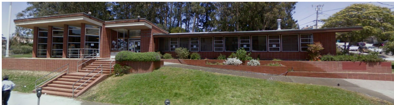
Parkside Branch Library, front façade, view north, 2008.
