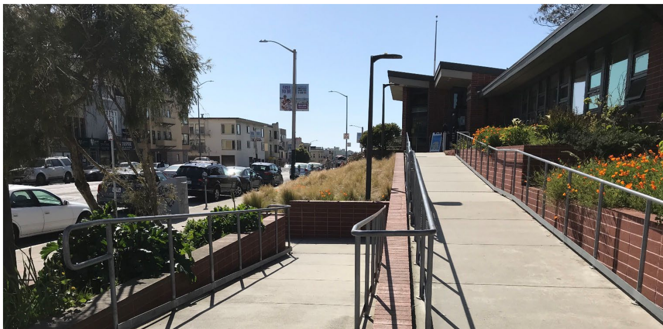
Parkside Branch Library, ramp at front, view west, 2023. Source: San Francisco Planning Department
