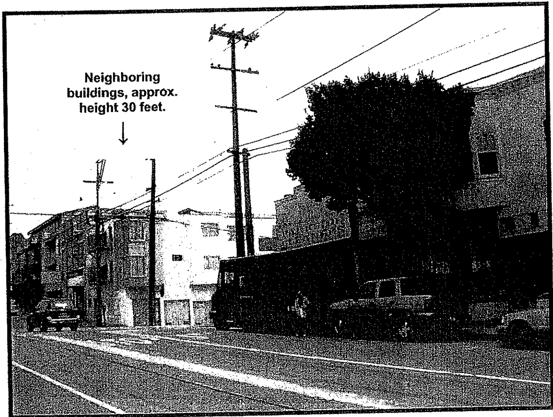
Viewing Southeasterly direction from Taraval Avenue, opposite Project Site.
