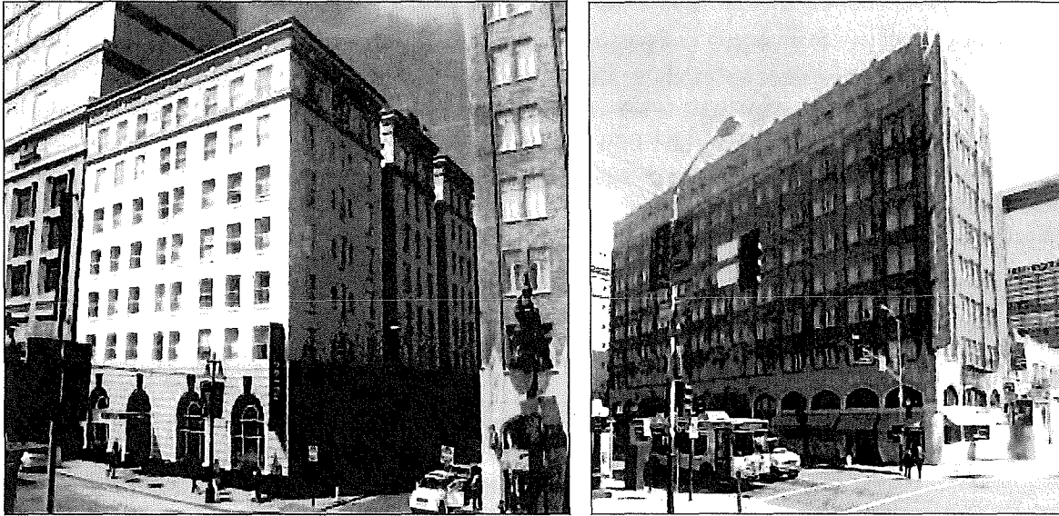
The Hotel Lankershim at left, and the Pickwick Hotel at right (Google Maps)
