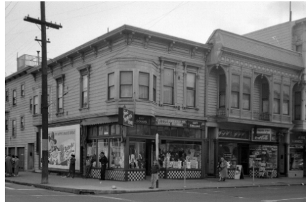
Figure 19: Galería de la Raza, 2851 24th Street. SF Assessor's archives, 1951 photo
